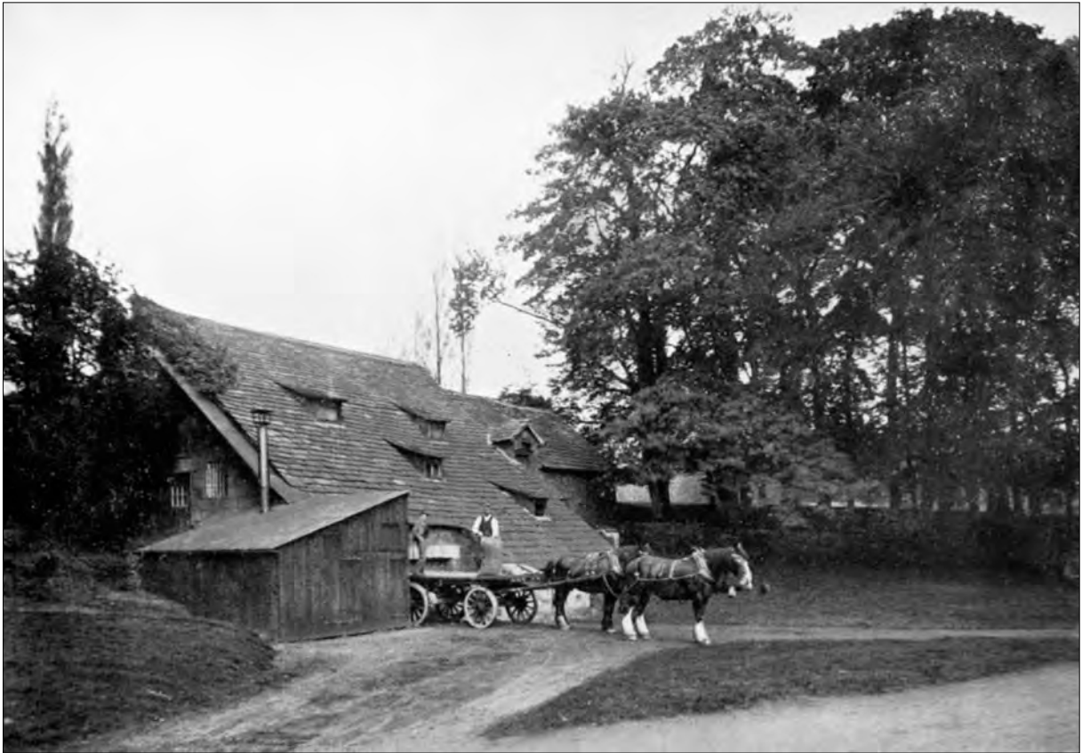
Figure 9: Nether Alderley Mill, c 1903 (Moss 1903).
