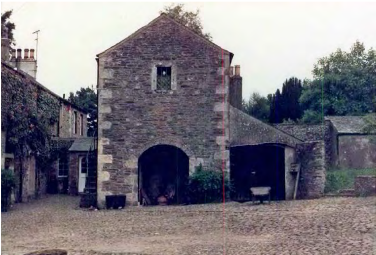
Figure 32: Building 2 from west, August 1987 (National Trust).
