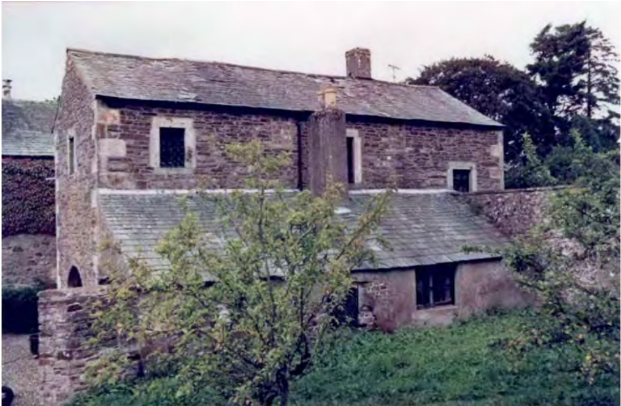
Figure 33: Building 2 from south, August 1987 (National Trust).
