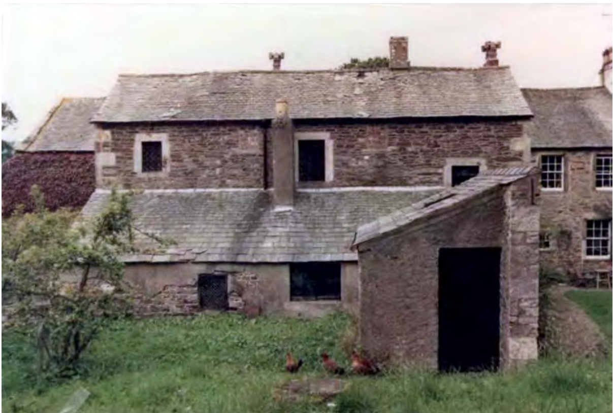
Figure 34: Building 2 from south, August 1987 (National Trust).
