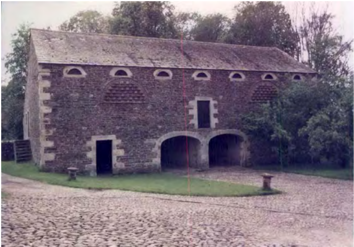
Figure 35: Building 3 from east, August 1987 (National Trust).
