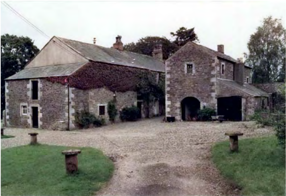
Figure 31: Buildings 1 and 2 from west, August 1987 (National Trust).
