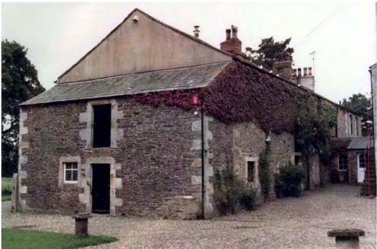
Figure 30: Building 1 from west, August 1987 (National Trust).
