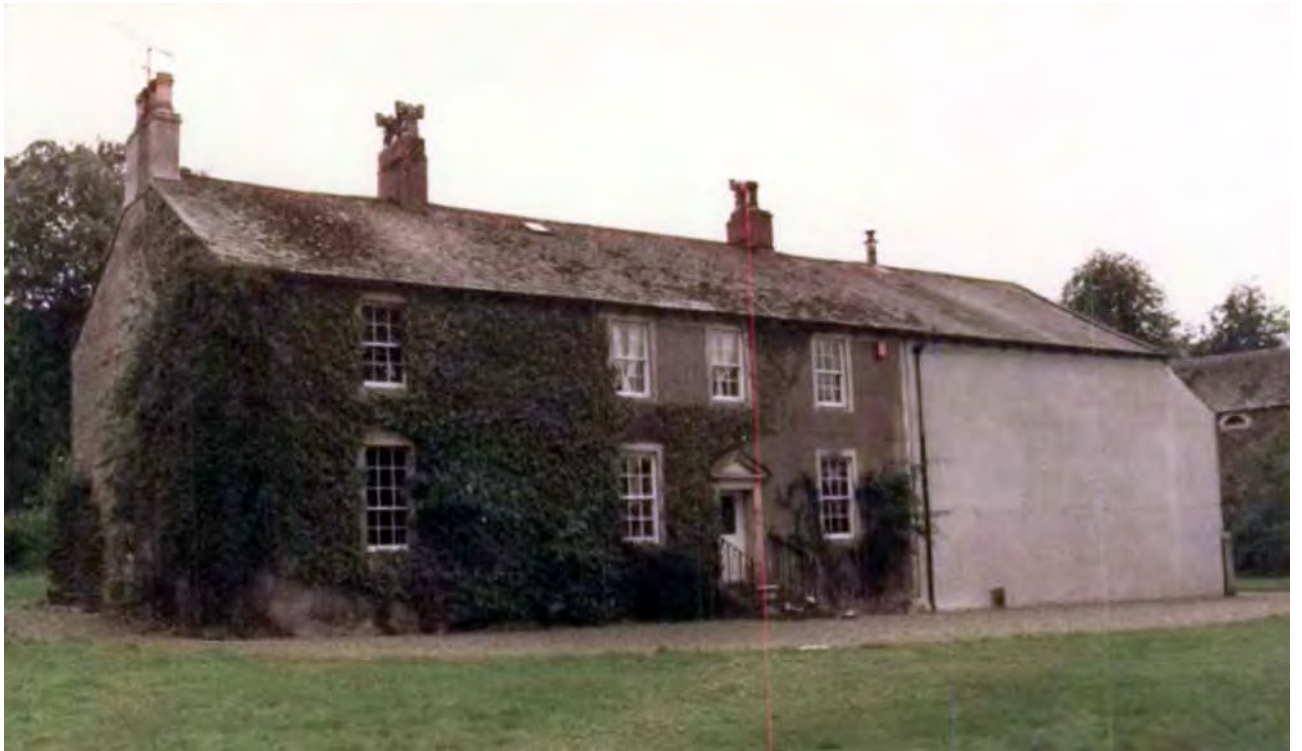
Figure 29: Building 1 from north, August 1987 (National Trust).
