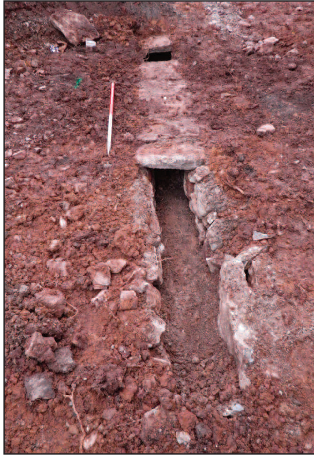
Plate 4 Close-up view of partially intact length of stone drain (108), looking north-east
