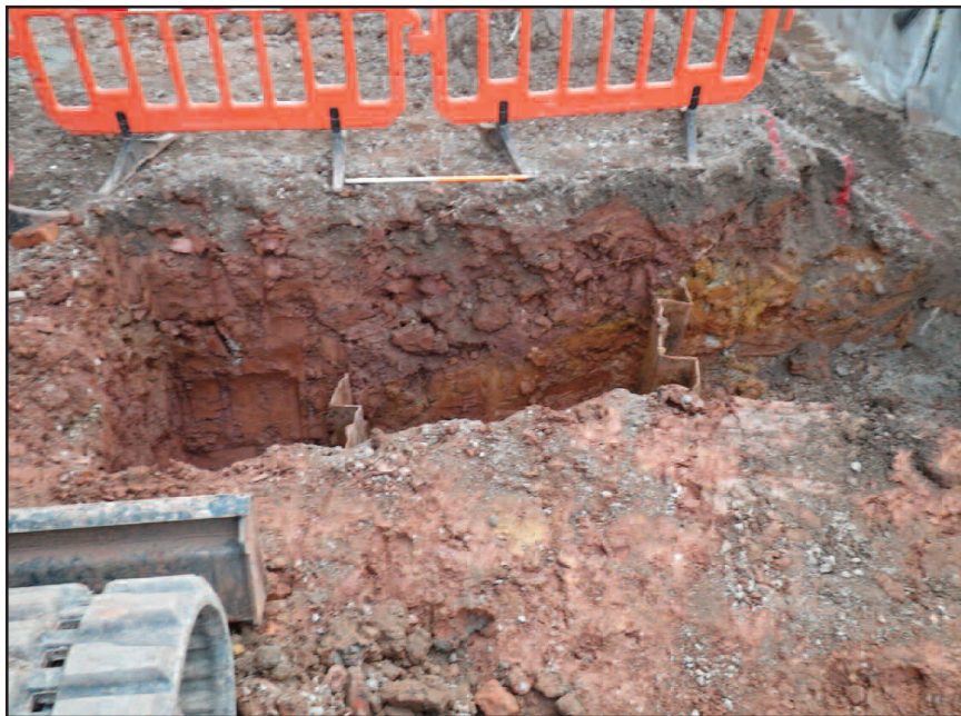
Plate 8 North-east facing section in foundation trench
