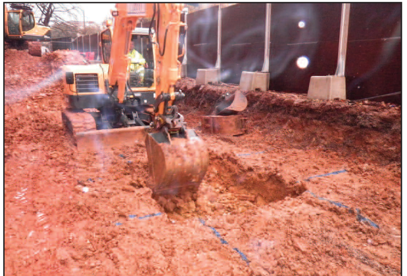
Plate 6 Excavating foundation pit, looking south-west
