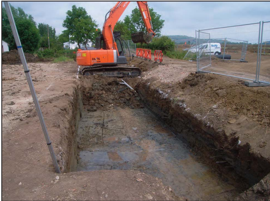
Plate 7 Looking north-east at the excavation of the trench for a new culvert to carry the flow of the South Brook beneath a new roundabout
