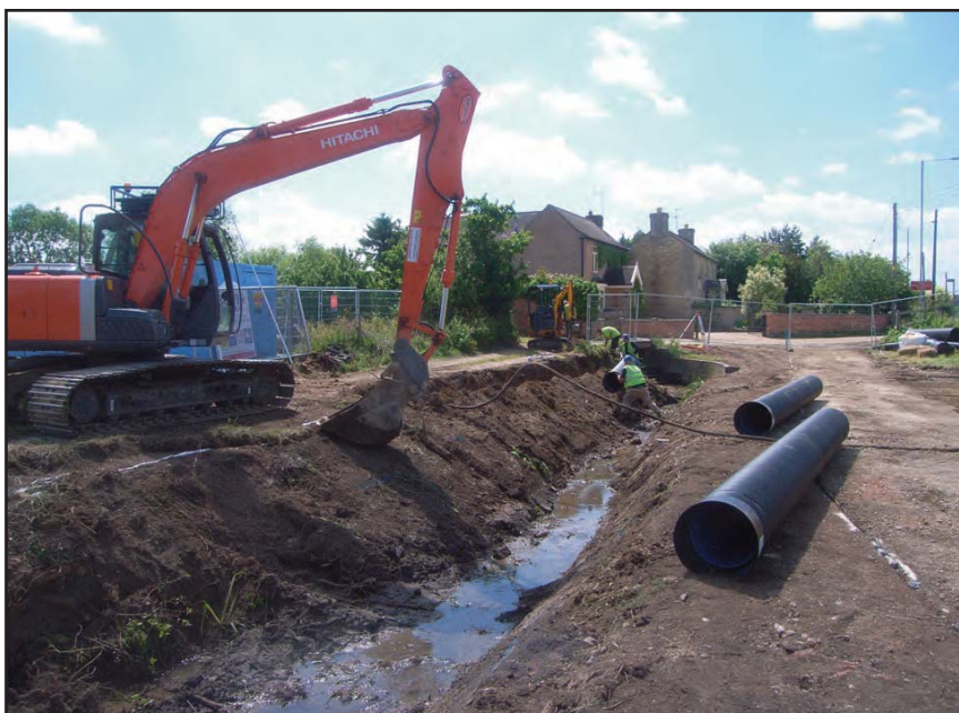
Plate 6 Excavation/pipe laying in progress on the line of the temporary stream diversion trench; looking south towards Nos. 56 & 58 Evesham Road
