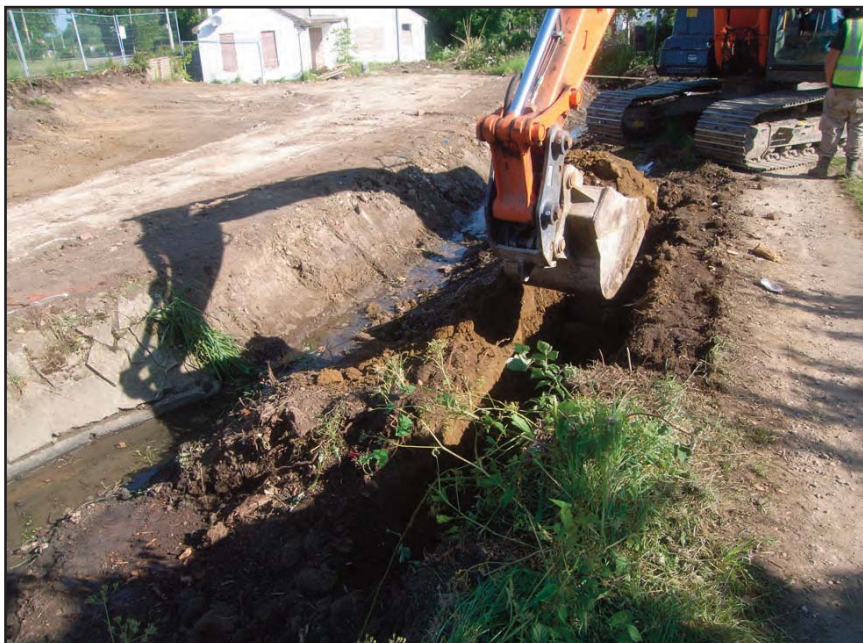
Plate 5 Excavation of stream diversion trench, looking north
