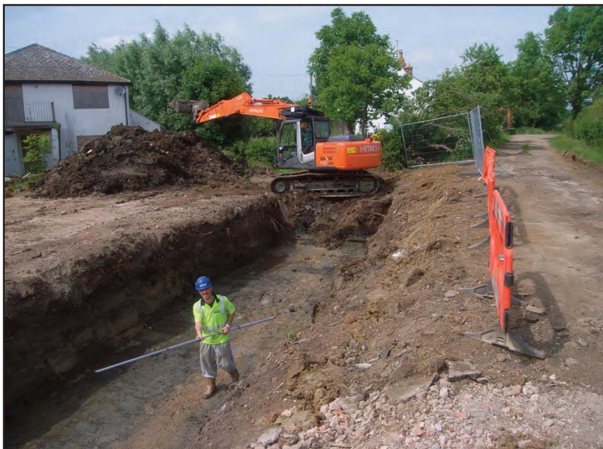
Plate 8 View north of the culvert trench, during excavation
