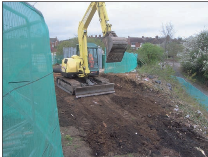
Plate 5 Excavation work underway (looking north) at the top of the embankment
