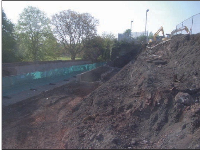
Plate 7 Looking south across the site during excavation/ground reduction work
