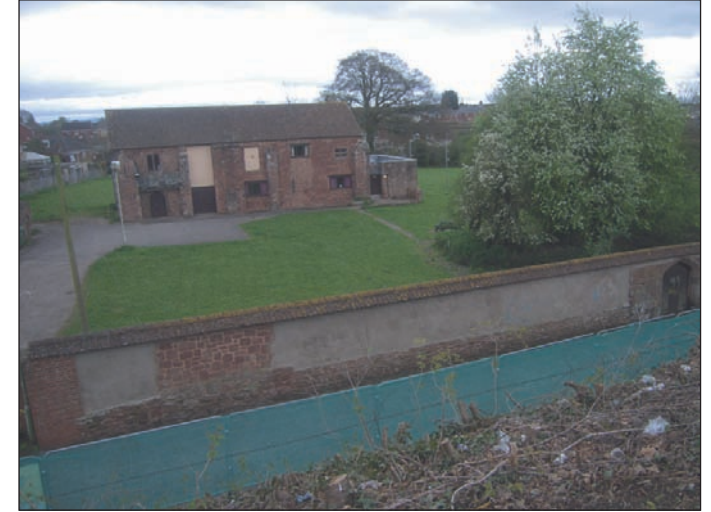
Plate 3 Looking east, from the top of the embankment, towards Polsloe Priory. Behind the boundary wall stands the two-storey former west range of the cloister, dating largely from c.1300
