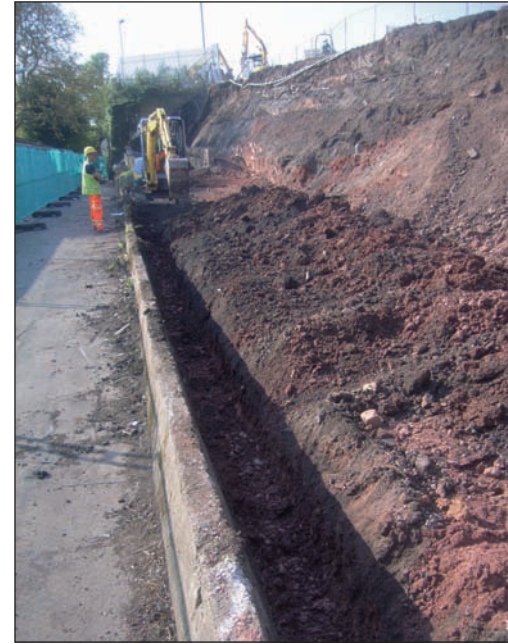
Plate 8 Looking south at excavation of foundation trench for new retaining wall
