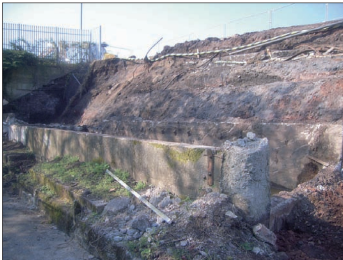
Plate 9 Looking south-west, from footpath, at remains of early 20th century water tank
