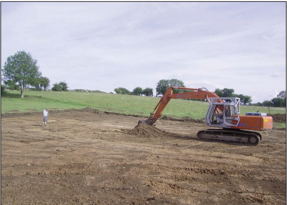
Plate 2 Stripping residual topsoil from the eastern end of the site, viewed from the north
