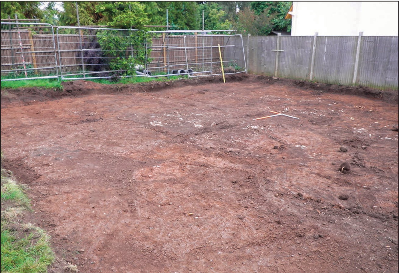
Plate 2 Reduced level excavation, undisturbed natural exposed, looking north
