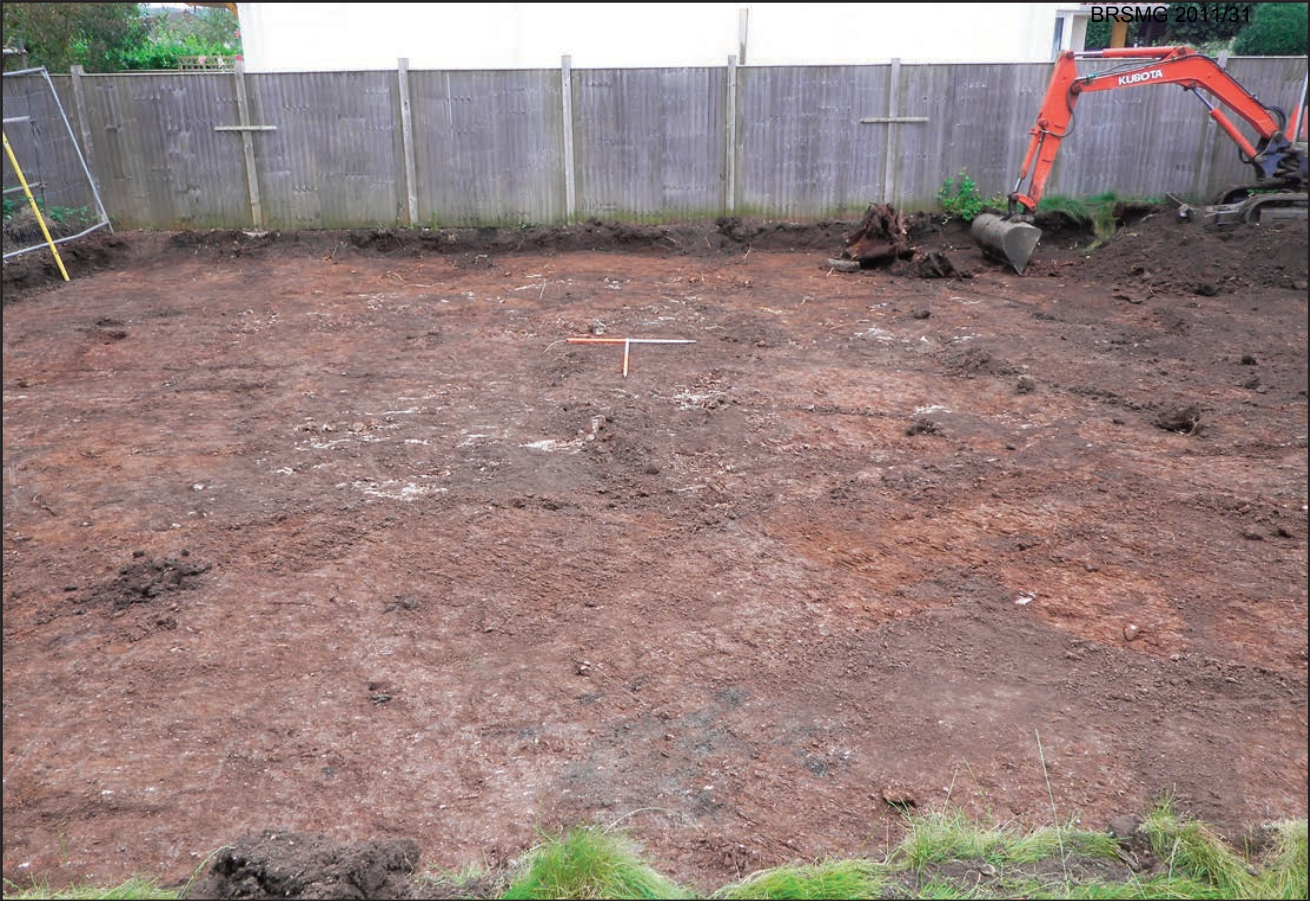
Plate 1 Reduced level excavation, undisturbed natural exposed, looking north-east
