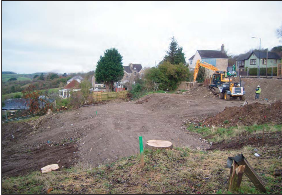
Plate 1 Ground level reduction work in progress, looking north-west
