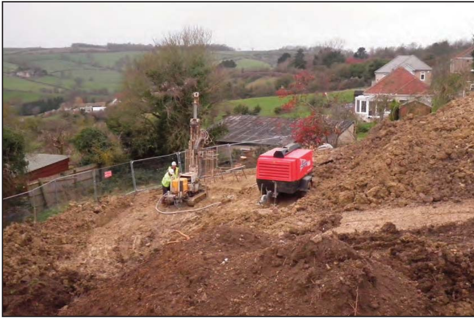
Plate 3 Investigative boreholes being drilled, looking south-west
