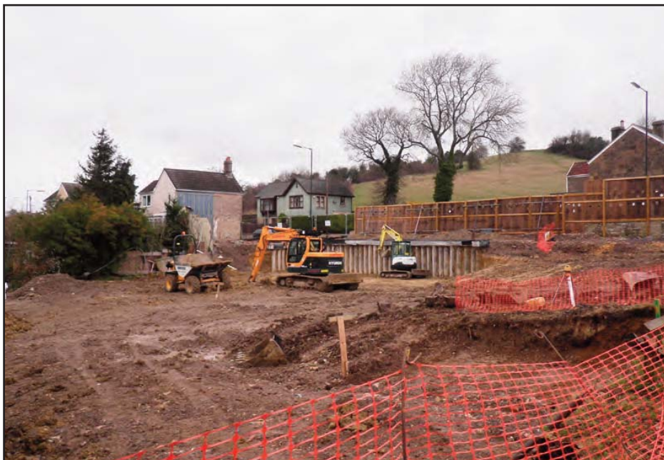
Plate 2 Excavation of foundation trenches for plots 2-5, looking north
