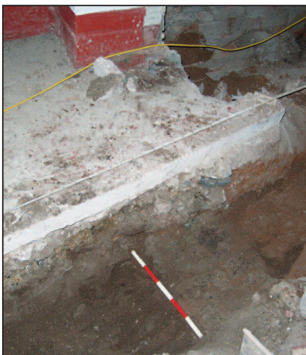
Plate 3 Foundations of internal partition-wall (119), viewed from the north-east
