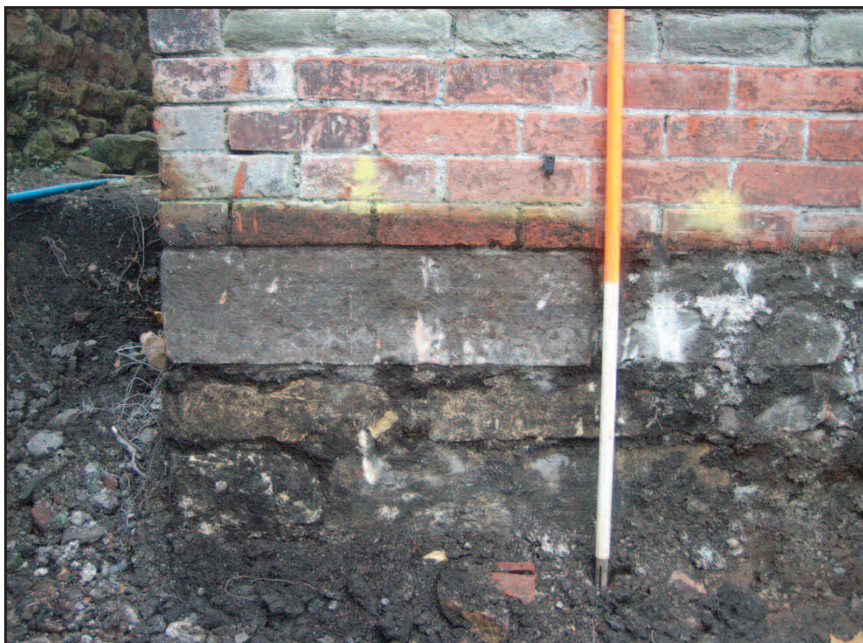
Plate 2 Foundations of the Old Gaol Stables (110)/(116), viewed from the east
