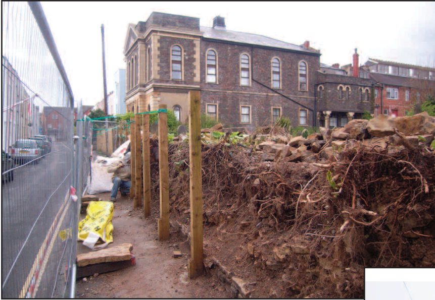
Plate 1 Rebuilding the boundary wall along Hebron Road, viewed from the north
