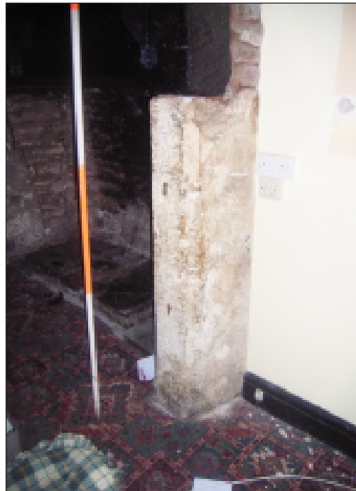
Plate 5 Stone slab, possible former gate-post, forming the north side of the fireplace in room 2, looking south-west
