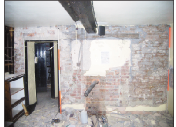
Plate 15 Stripped south elevation (east end) of room 2, looking south
