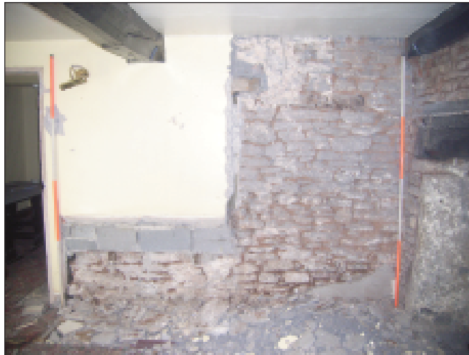
Plate 14 Stripped south elevation (west end) of room 2, looking south
