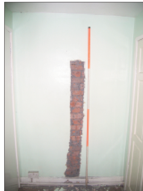
Plate 28 Stripped area in room 6, 1st floor exposing brickwork, looking north
