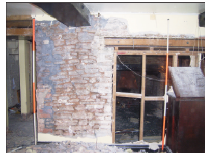
Plate 12 Stripped north elevation (east end) of room 2, looking north
