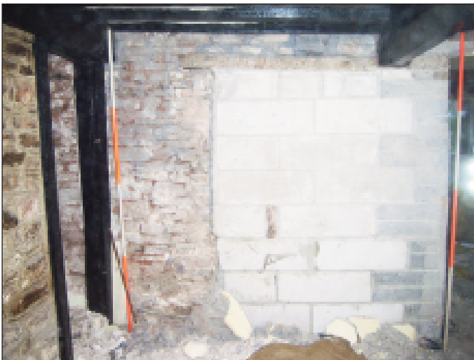
Plate 17 Stripped east elevation of room 1, looking east
