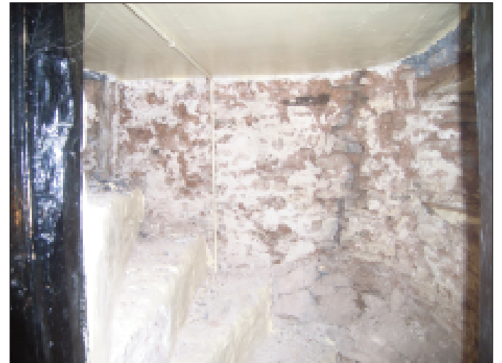
Plate 18 Stripped stairwell in north-east corner of room 1, looking north
