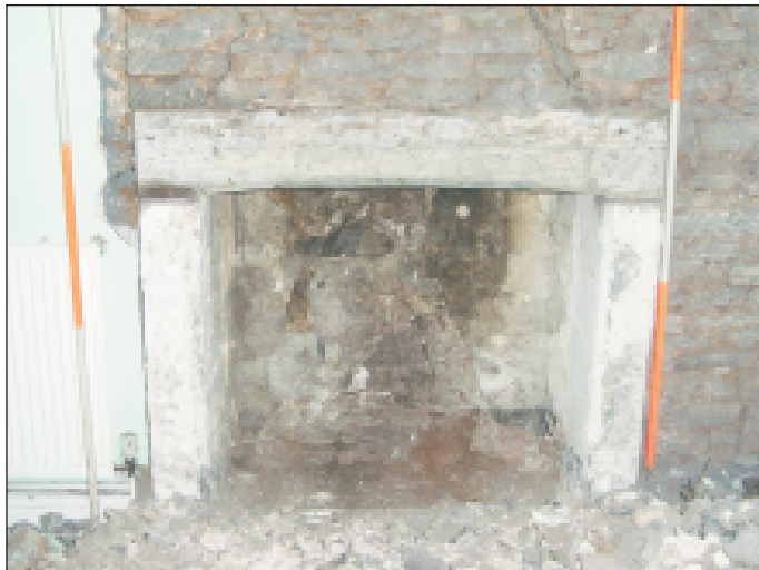
Plate 22 Original fireplace in room 4 opened up, looking east
