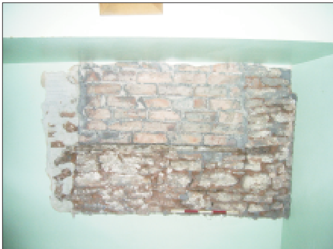
Plate 25 Stripped area in room 3, 1st floor exposing a blocked opening, looking north
