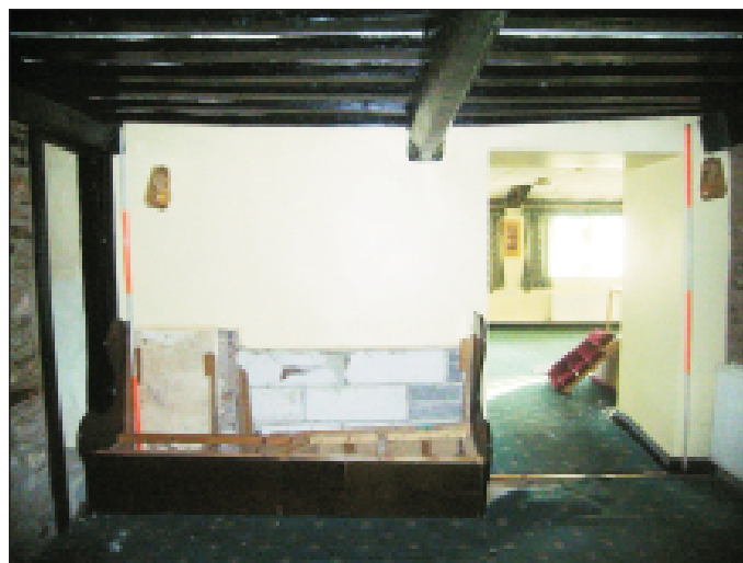
Plate 8 East internal elevation of room 1 of the historic core ground floor, looking east
