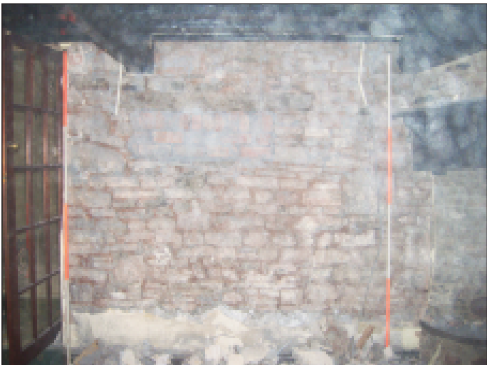
Plate 16 Stripped west elevation of room 1, looking west
