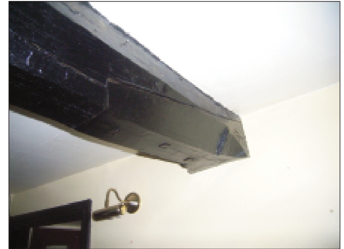
Plate 6 North end of room 2 beam with carved stops, looking north-west
