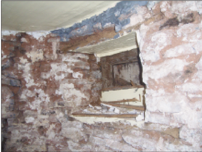
Plate 19 Original window in wall of stairwell, looking north-east
