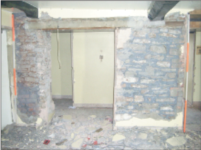
Plate 13 Stripped north elevation (west end) of room 2, looking north
