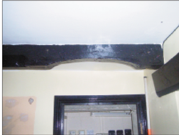
Plate 2 Cut in west beam of room 2 for a former opening, looking west
