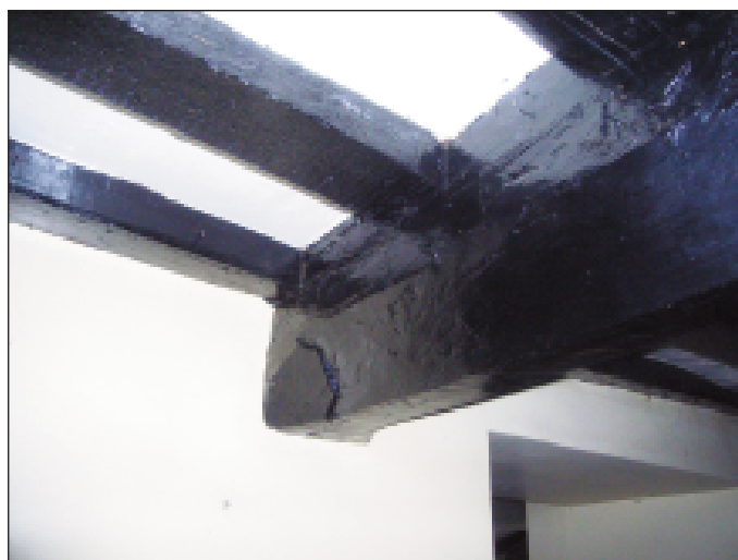
Plate 11 East end of room 1 central beam with carved stops, looking south-east
