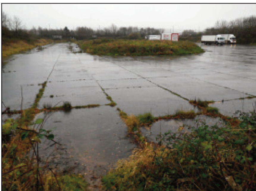
Plate 6 Hangar site, concrete apron now used for HGV driver training, looking south
