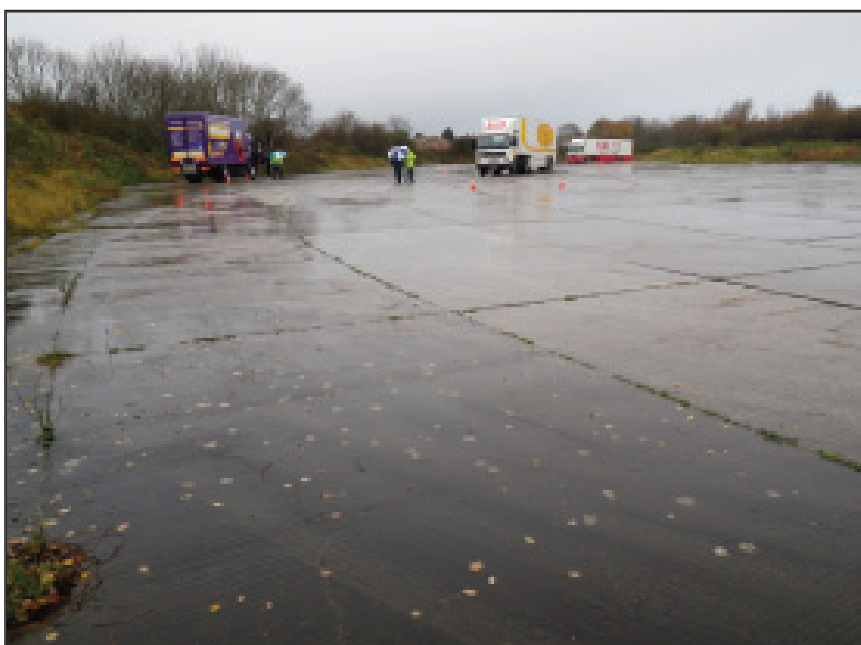
Plate 5 Hangar site, concrete apron now used for HGV driver training, looking north
