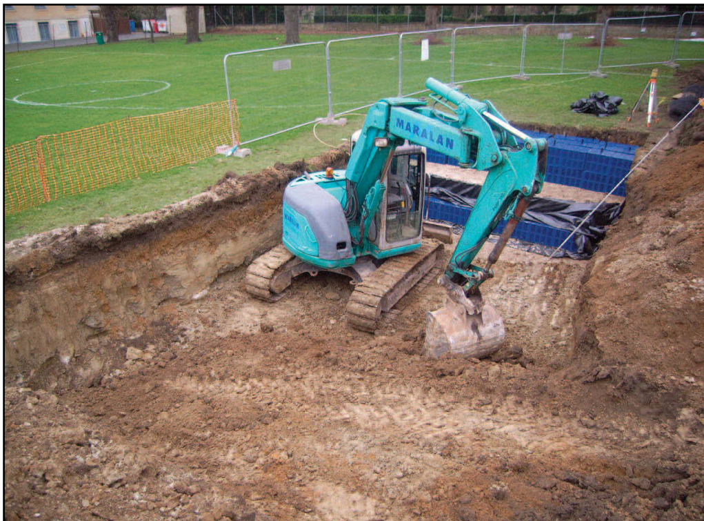
Plate 4 Excavating the attenuation tank, viewed from the south-west
