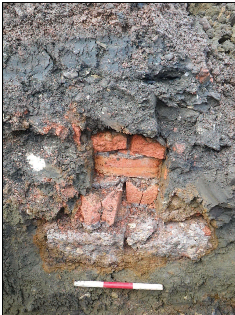
Plate 2 Typical section of 1940s hutment foundations
