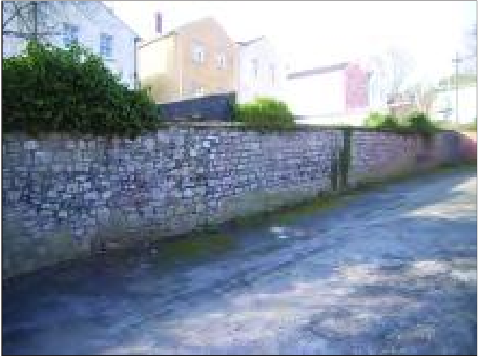
Plate 22 Original south-west boundary wall of the site, looking west
