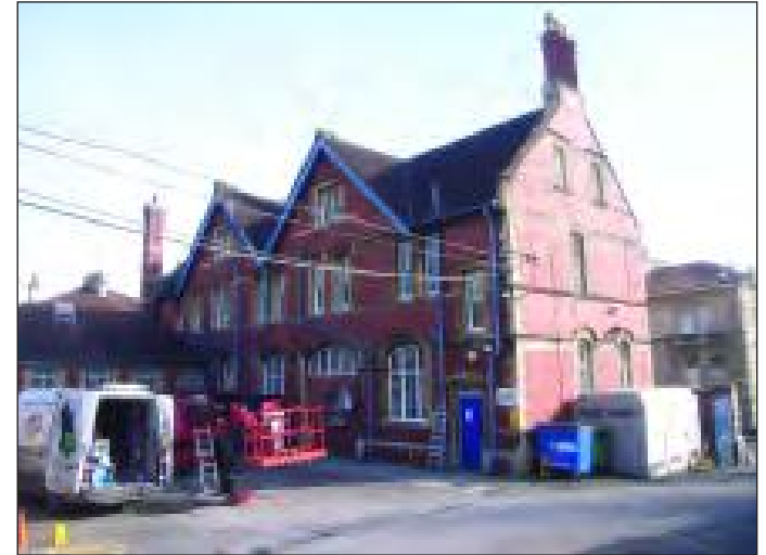
Plate 3 Rear of the main building of Redland Police Station, looking east
