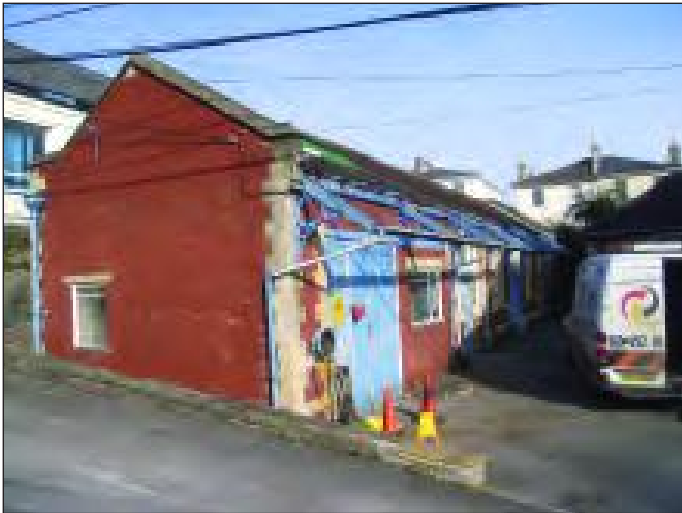
Plate 10 'Stable' block of Redland Police Station, looking north
