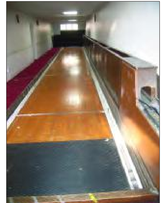
Plate 18 Skittle alley in the recreation block, looking north-west
