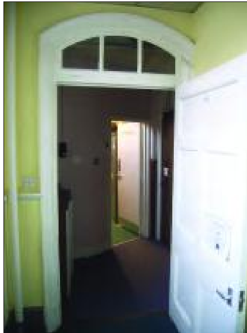
Plate 5 Original doorway on ground floor of the main building, looking north-east
