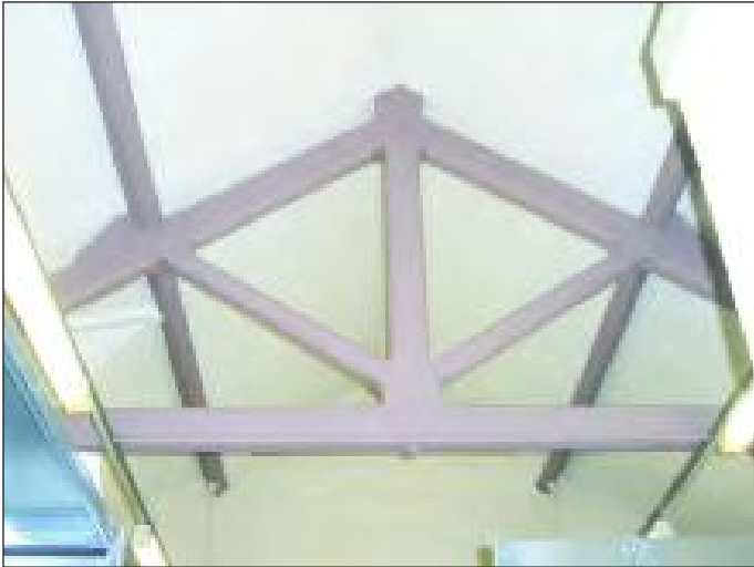
Plate 13 King-post roof truss of the 'stable' block, looking north-east
