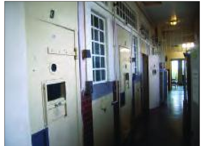
Plate 6 Cells area of the main building, looking south-east
