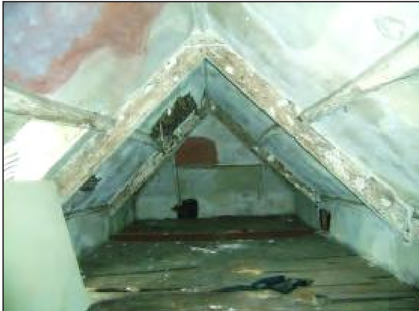
Plate 16 Attic space above Swetnam wing, showing original roof timbers, looking north-west
