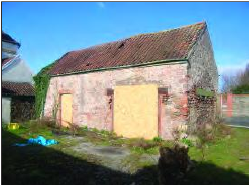
Plate 7 Detached outbuilding (inaccessible at time of site visit) looking north- west
