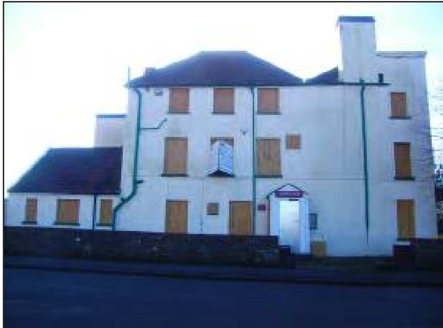
Plate 10 Old Ferry House frontage, note repositioned ground floor windows and door, looking south-east
