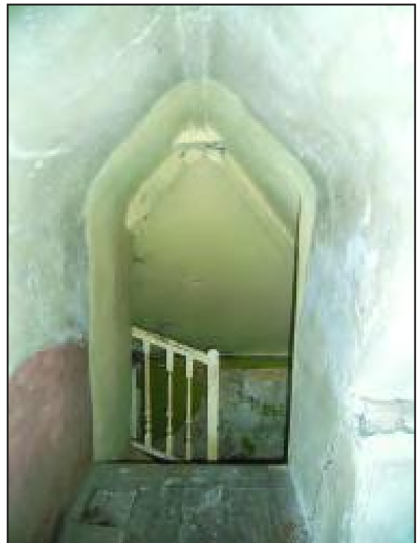
Plate 15 Stairway to attic space in Swetnam wing, looking north-east
