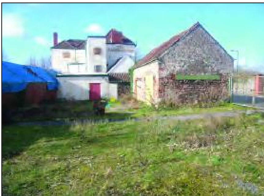
Plate 6 Looking south-west from yard area towards rear of Lamplighters buildings, (1970s service wing and extension in centre of photo)
