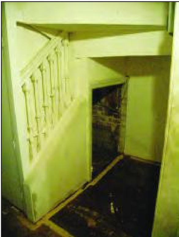
Plate 14 Second floor in Swetnam wing showing stairway to attic space truncated by 1970s service-wing, looking south-east
