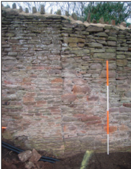
Plate 5 Central area of the wall segment showing vertical 'break', interior face, looking west
