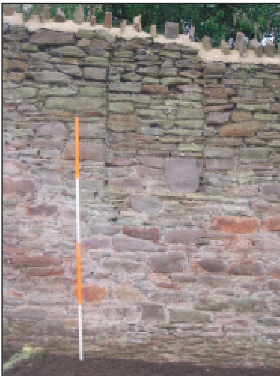
Plate 8 Northern blocked-in Opening B, interior wall face, looking west
