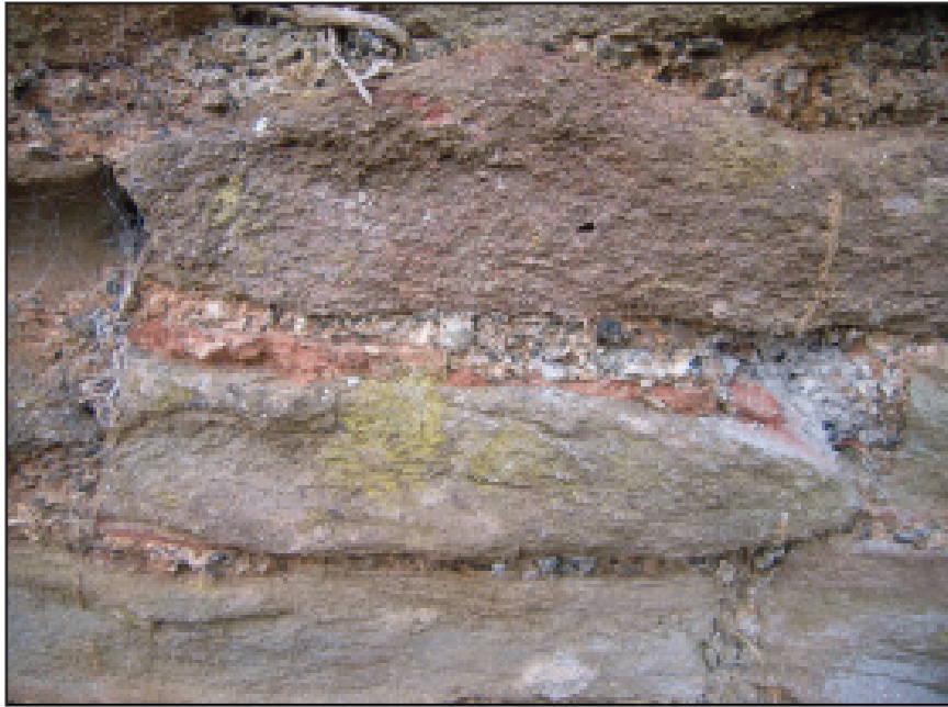
Plate 10 Mortar details on interior wall, showing 'scraped out' pinkish mortar and later ashy mortar re-pointing
