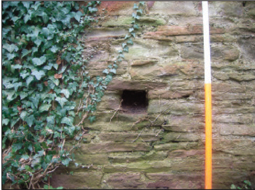
Plate 7 Drainage hole on exterior wall face, looking east
