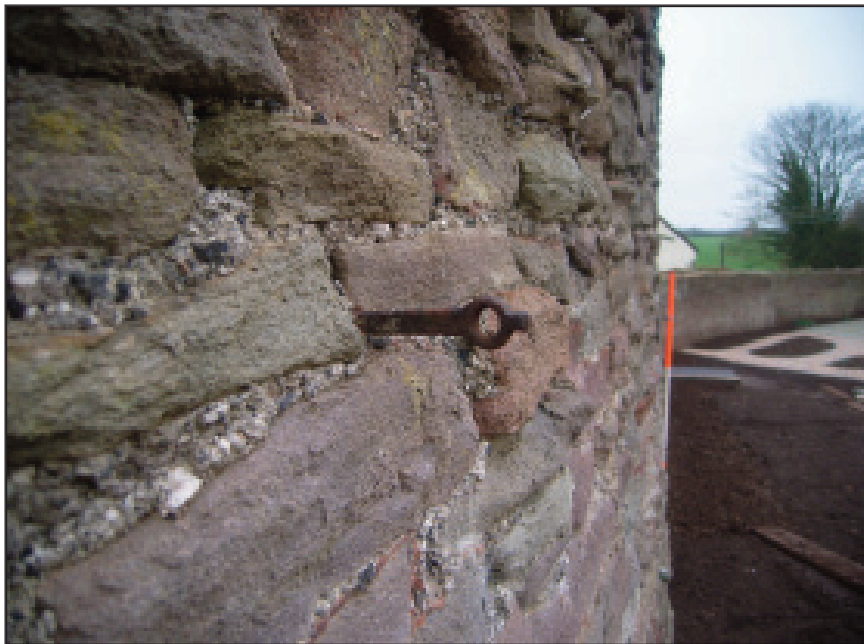
Plate 11 Example of iron trellis pin set into ashy mortar, looking north
