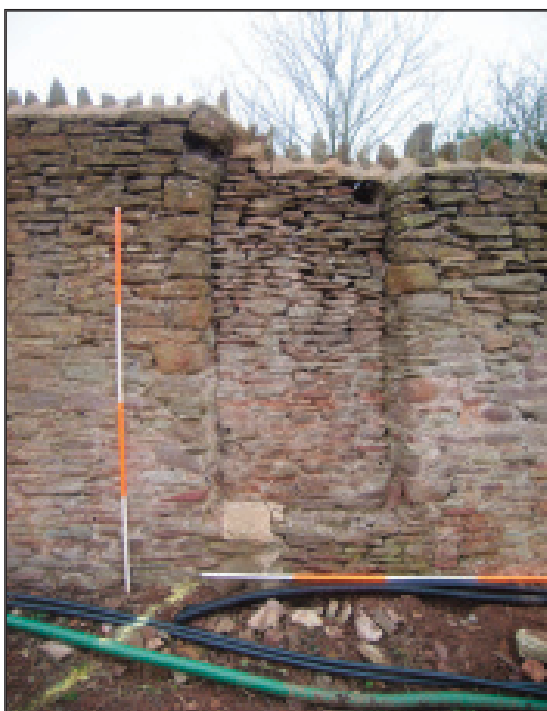
Plate 3 Southern blocked-in Opening A, interior face, looking west
