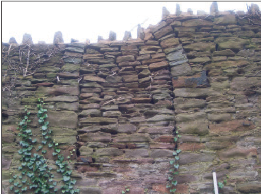
Plate 4 Southern blocked-in Opening A, exterior face, facing east
