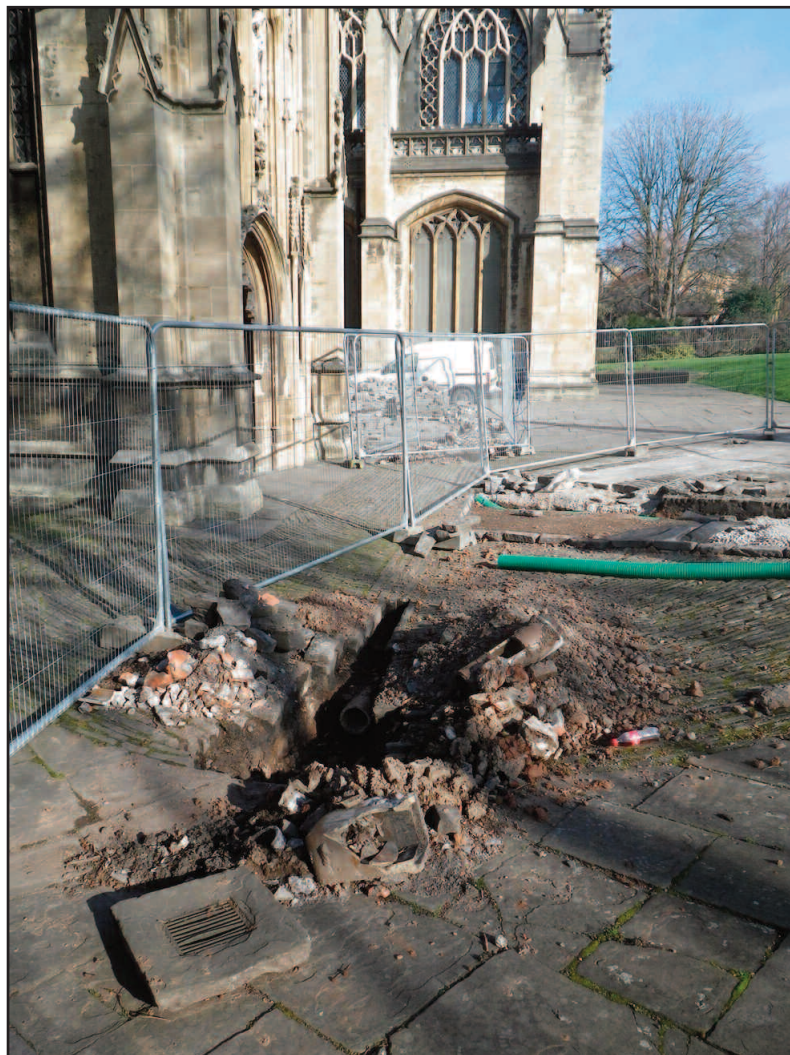
Plate 2 Trenches adjacent to southern porch for new drainage gully pots
