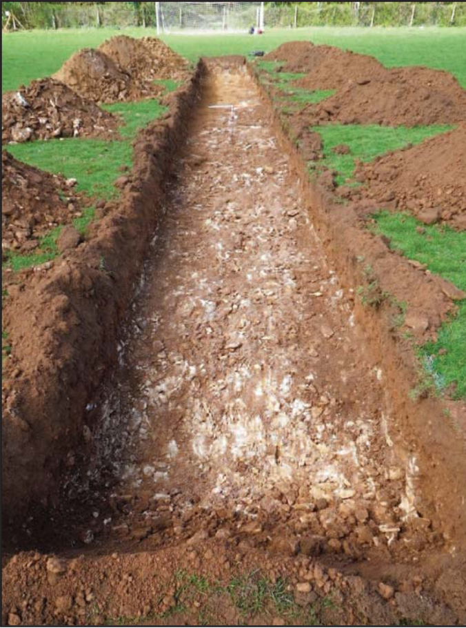
Plate 1 Trench 1, viewed from the east
