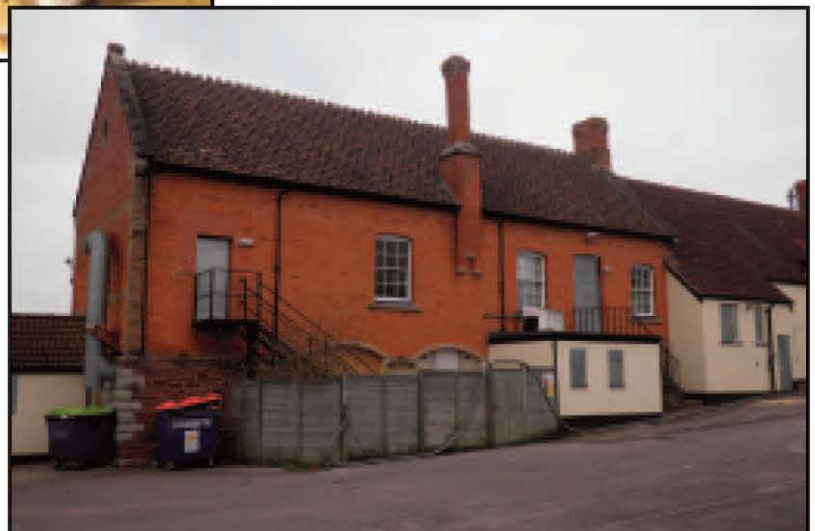
Plate 8 East-facing elevation of Assembly Room / Carriage-shed building – looking west
