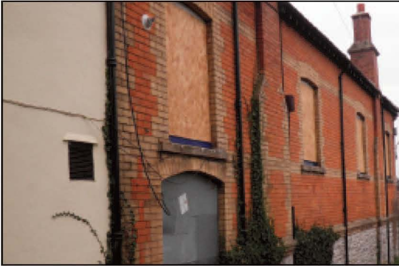
Plate 9 West-facing elevation of Assembly Room / Carriage-shed building – looking south-east from footpath
