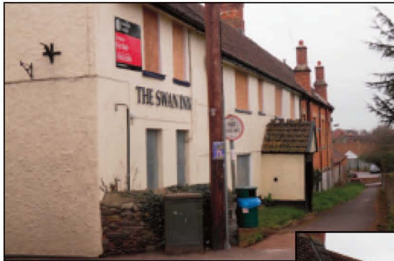
Plate 1 West-facing elevation of the Swan Inn, looking south-east
