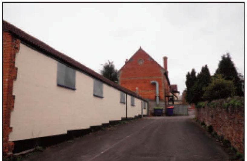
Plate 12 East-facing elevation of former stables – looking north-west
