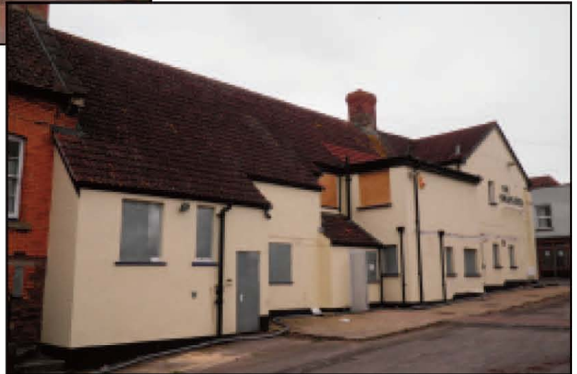
Plate 2 East-facing elevation of the Swan Inn, looking north-west
