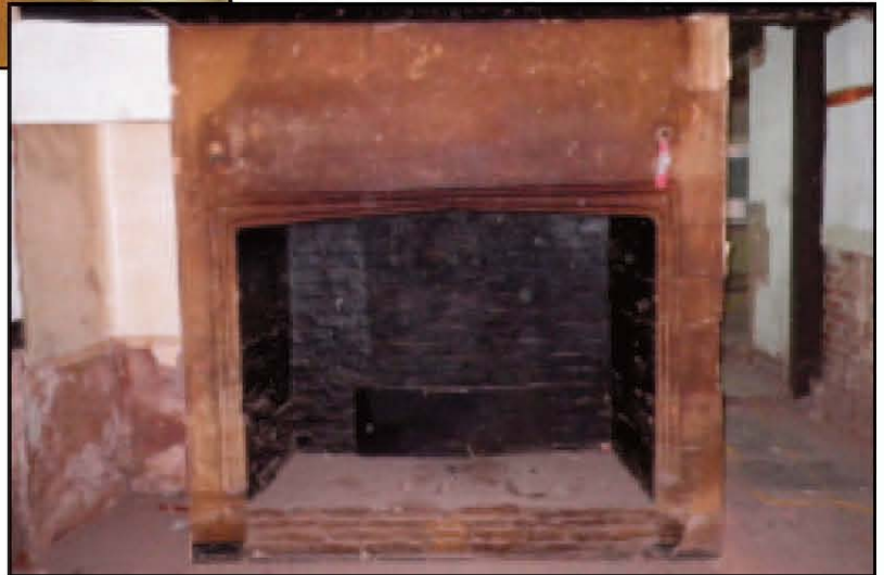
Plate 6 Close-up view of fireplace – looking north
