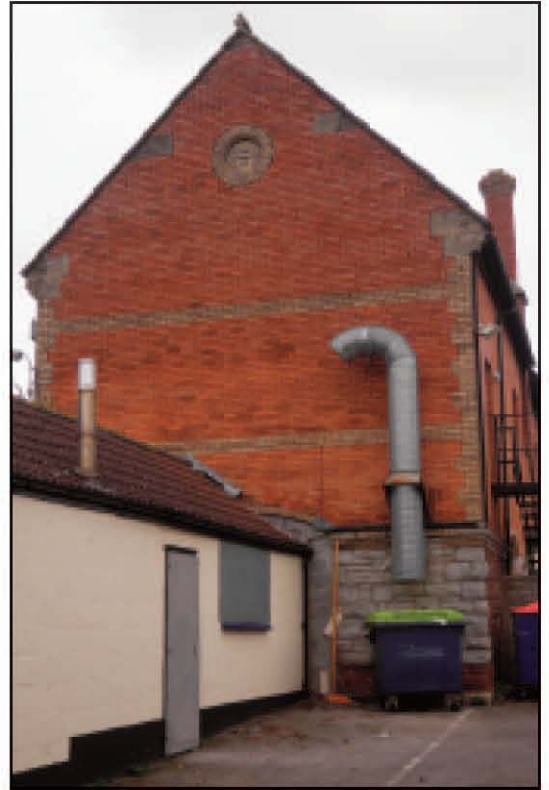
Plate 10 South-facing elevation of Assembly Room / Carriage-shed building – looking north
