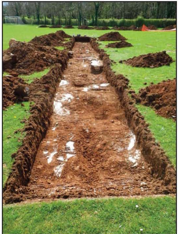
Plate 5 Trench 5, viewed from the north-east
