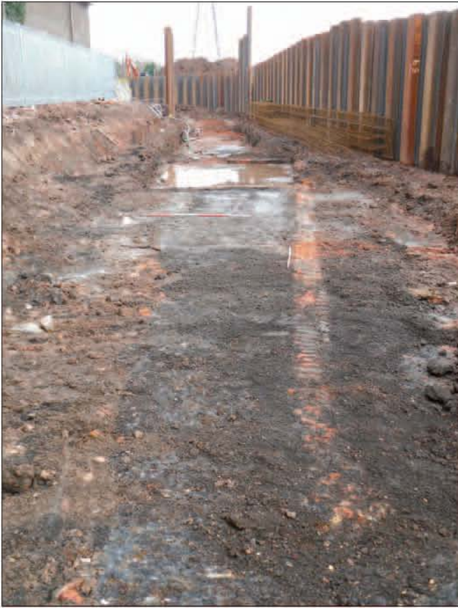
Plate 4 Brickworks structures 703-6, looking north-east
