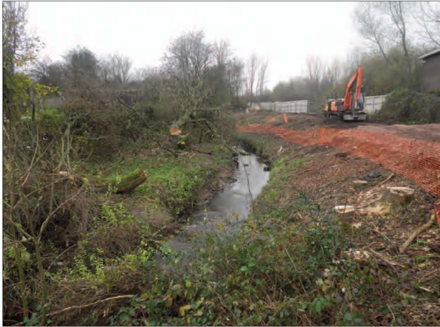
Plate 1 The Stonehouse Brook during initial clearance work, looking south-west
