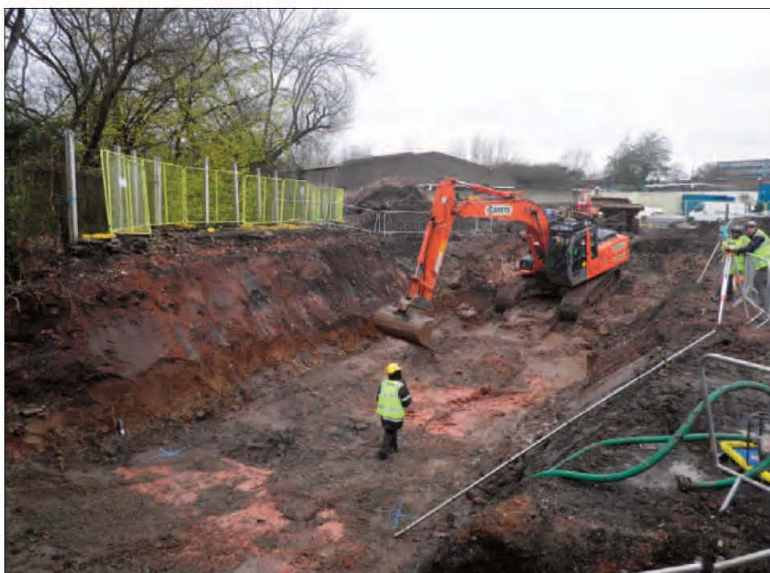
Plate 3 Permanant diversion of the Stonehouse Brook, looking south-west
