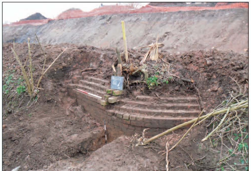
Plate 9 Tramway bridge abutment 900, looking south-east
