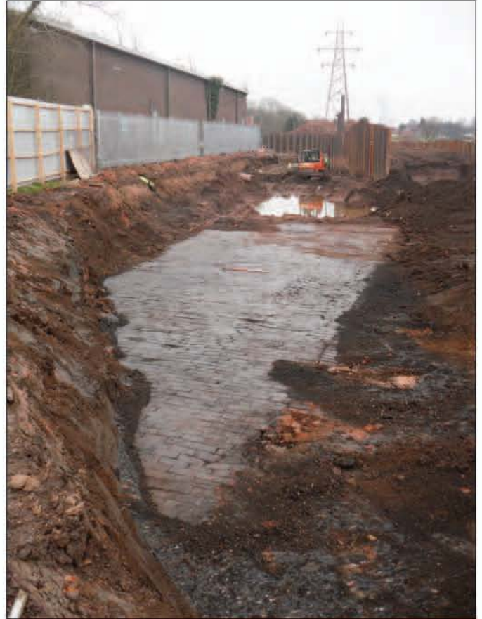
Plate 5 Brickworks structures 718-9, looking north-east
