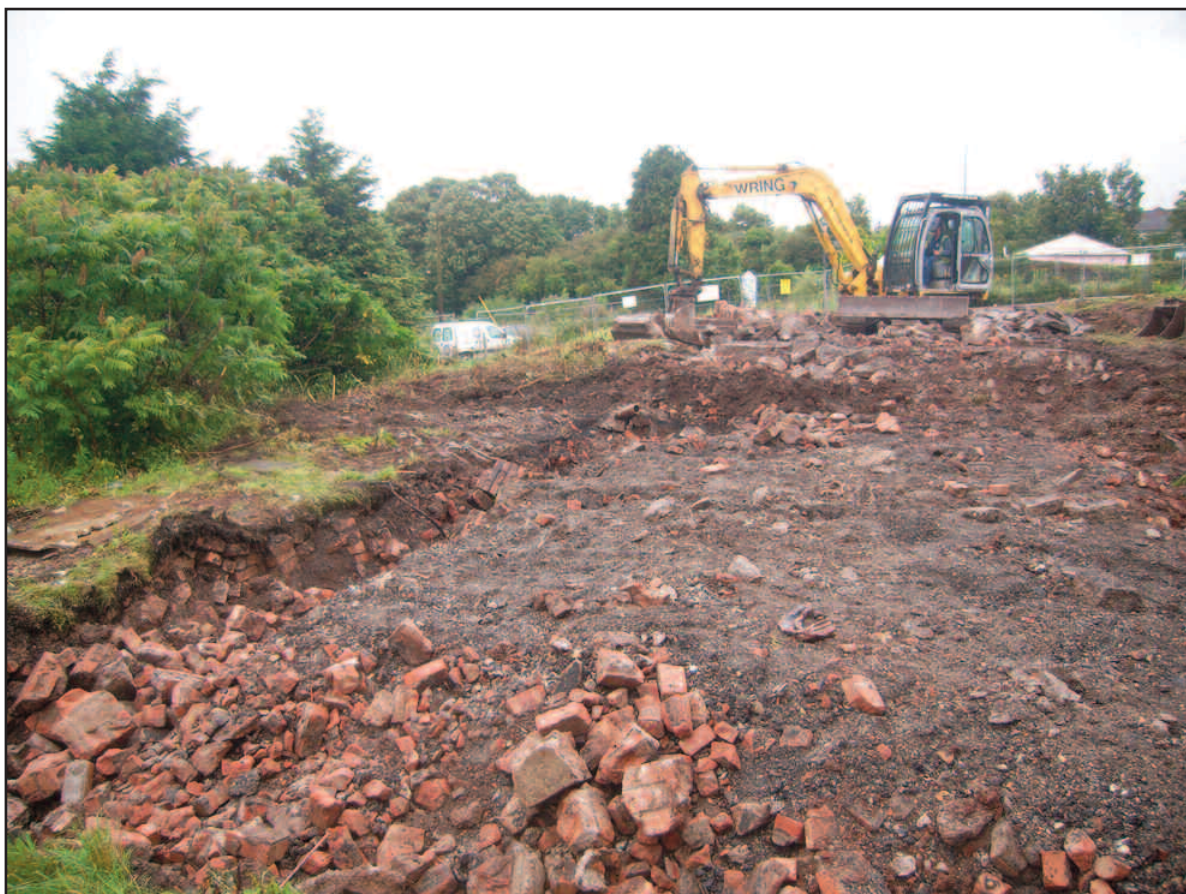
Plate 2 Rubble core (101) of prefabricated house foundations, viewed from the south-west
