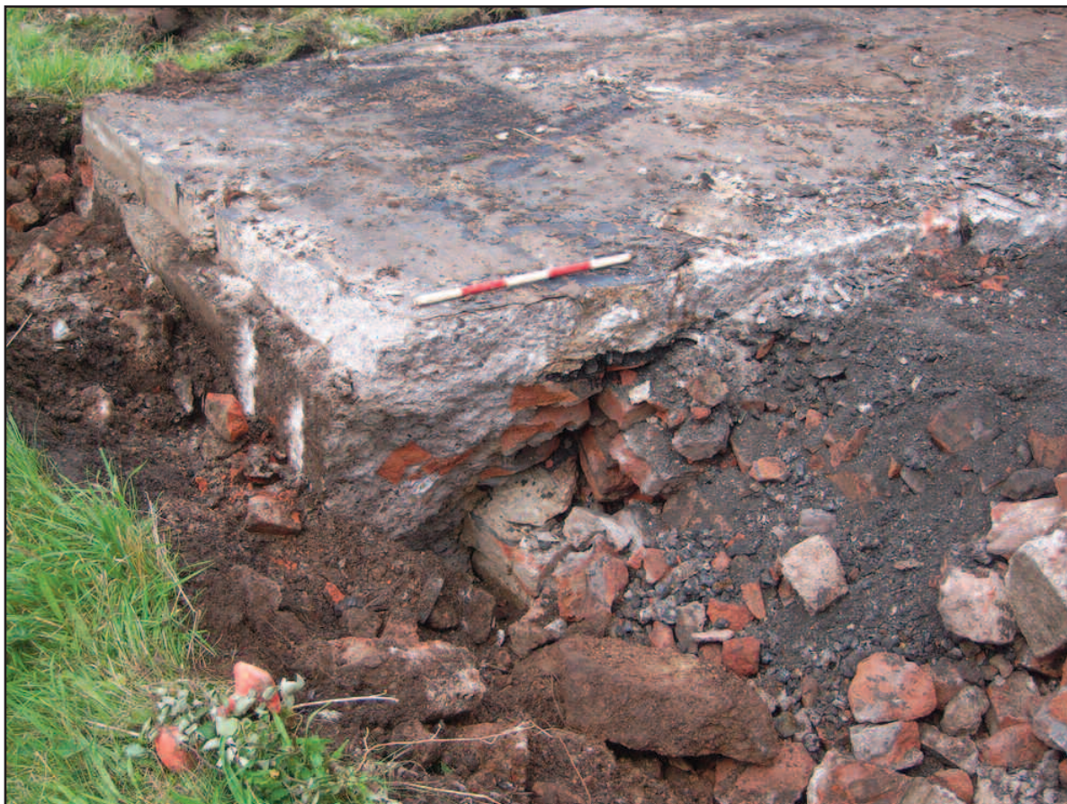
Plate 1 Concrete foundation (102) of 1940s prefabricated house, showing brick-rubble (101) to the right and brick-rubble (104), to the left. Viewed from the south
