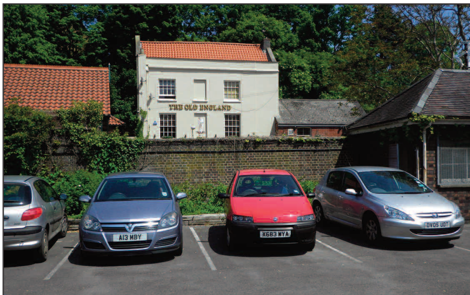
Plate 1 Boundary wall on the north-east side of the study area, with the Old England Public House visible in the background, looking north-east
