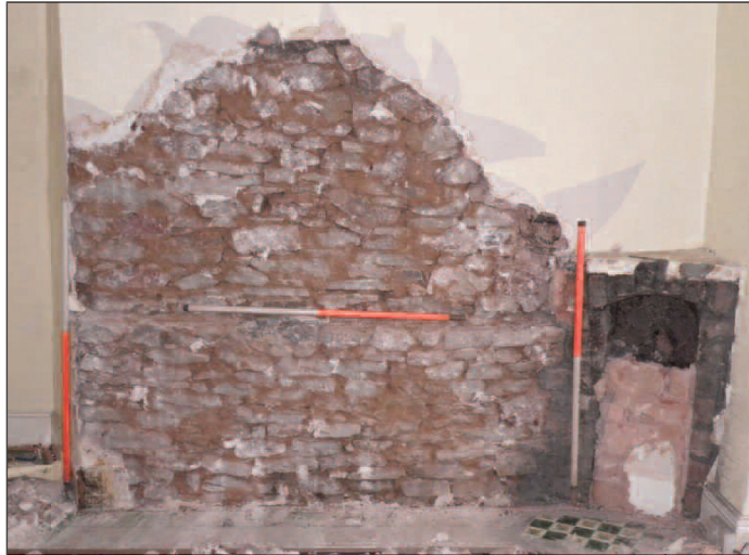
Plate 14 Stripped chimney breast forming east wall of the upstairs living area, looking east
