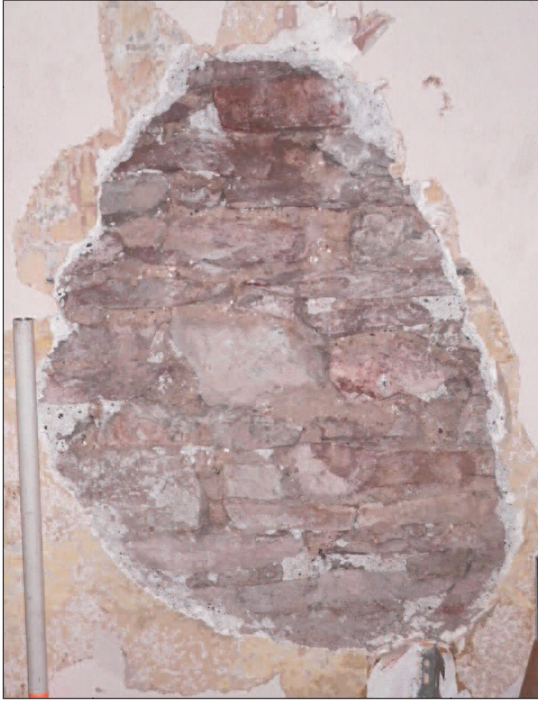
Plate 7 North wall of the front east bedroom, looking north
