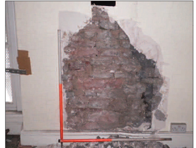
Plate 12 South wall of the upstairs living area, looking south
