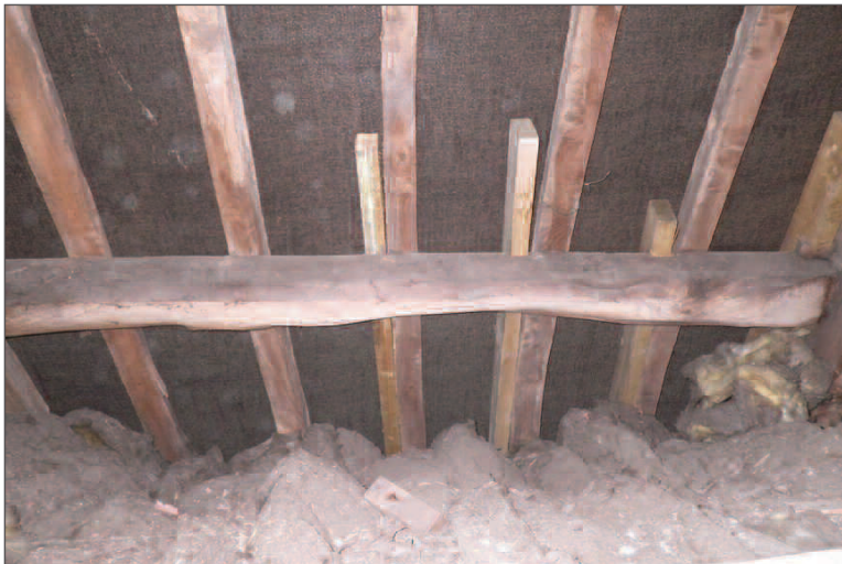
Plate 16 Purlin and rafters of the south pitch of the roof, looking south
