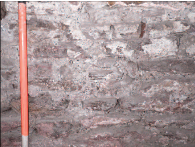
Plate 4 Exposed stonework in the central bar area north wall, looking north
