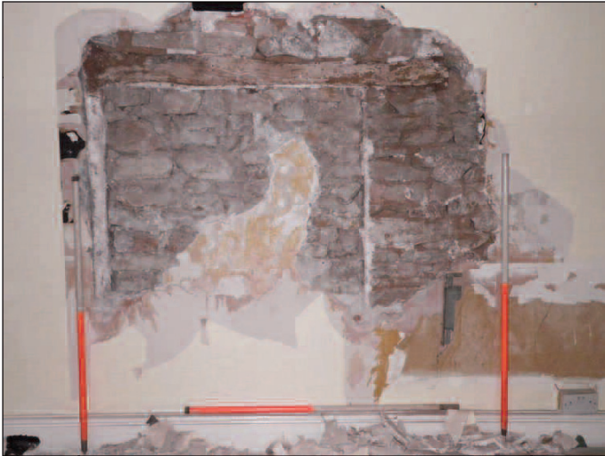
Plate 13 North wall of the upstairs living area, looking north
