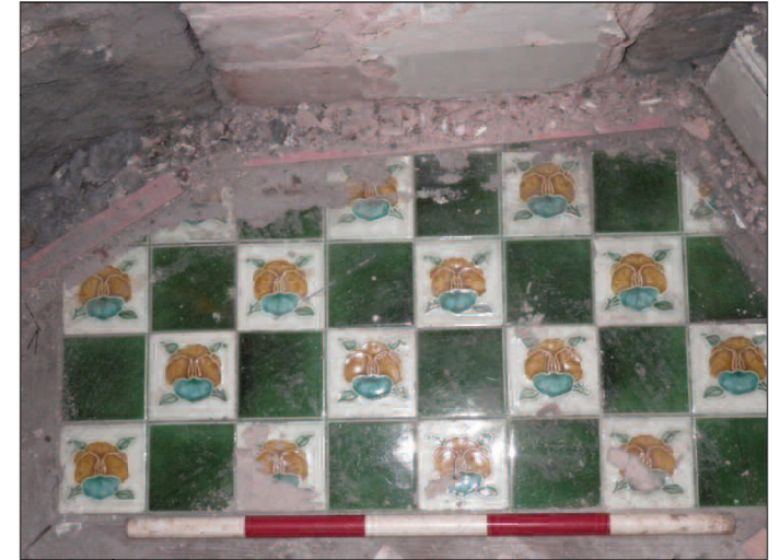
Plate 15 Glazed tiles forming the small hearth of the small inserted fireplace in the upstairs living area, looking south-east
