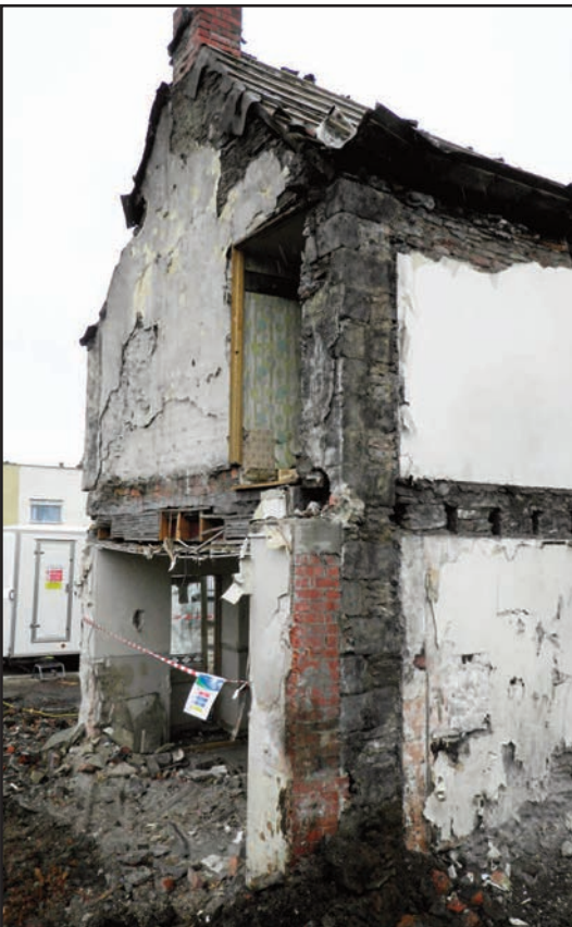
Plate 7 Slag block quoins in east end elevation of the historic core of the public house, looking south-west
