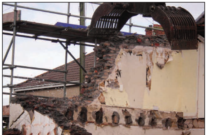
Plate 8 West end elevation during demolition, looking north-west
