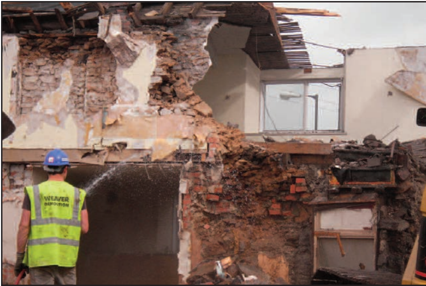
Plate 1 Western half of the central wall, clay-bonded stonework visible with later additions, looking north-east
