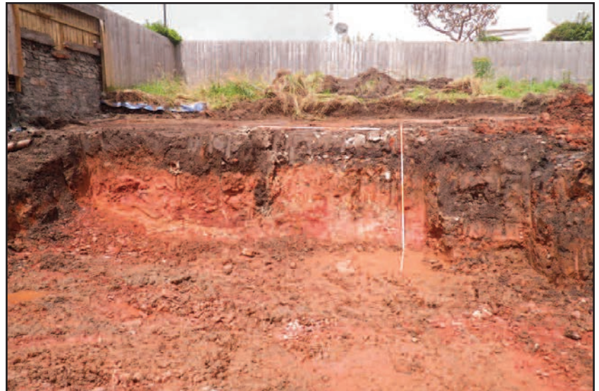
Plate 21 North section of cellar extension, looking north
