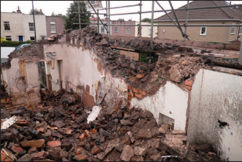
Plate 5 West end elevation during demolition, looking south-west
