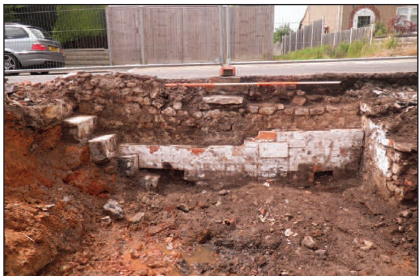
Plate 12 West elevation of the original cellar, looking west
