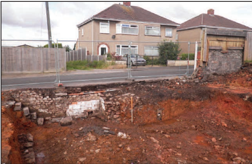
Plate 15 West section of the cellar area, looking north-west
