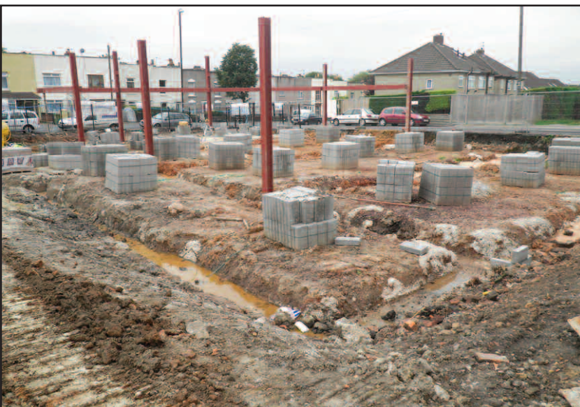
Plate 25 General view of the site during construction, looking south-west
