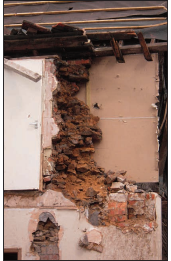
Plate 2 Western half of the central wall, clay-bonded stonework visible, looking north
