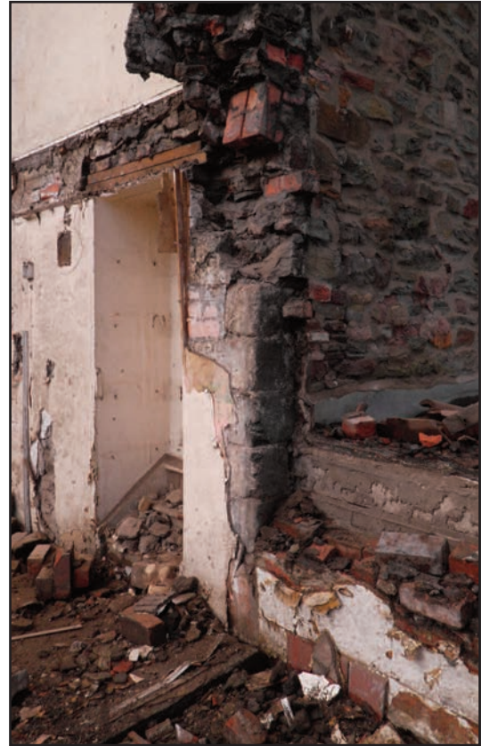
Plate 6 Slag block quoins in north elevation, looking south-west
