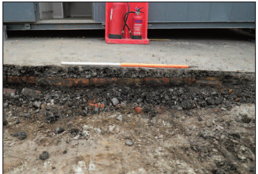
Plate 24 Section of brick foundations of the 19th-century out-houses demolished in 1971, looking east
