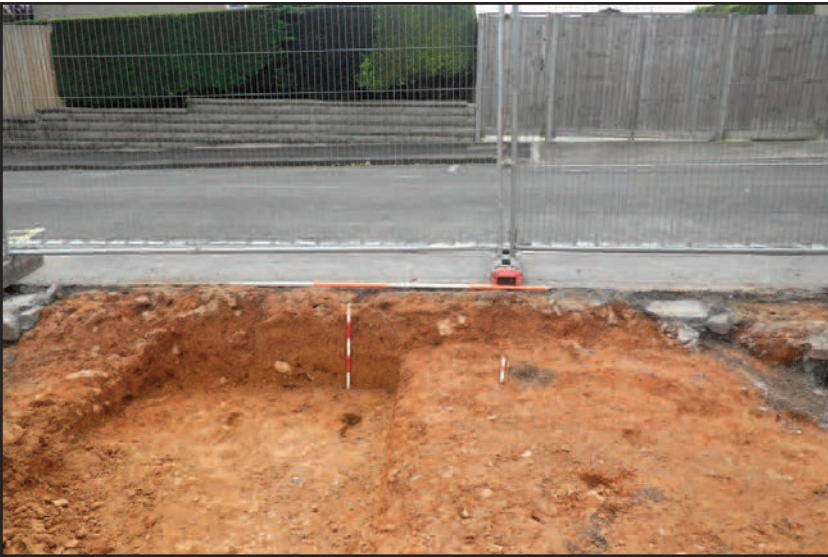
Plate 9 Remnant of west elevation footings, with truncated pit (1003), looking west
