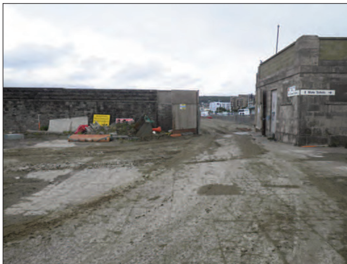
Plate 26 New entrance knocked through the north sea wall, looking north
