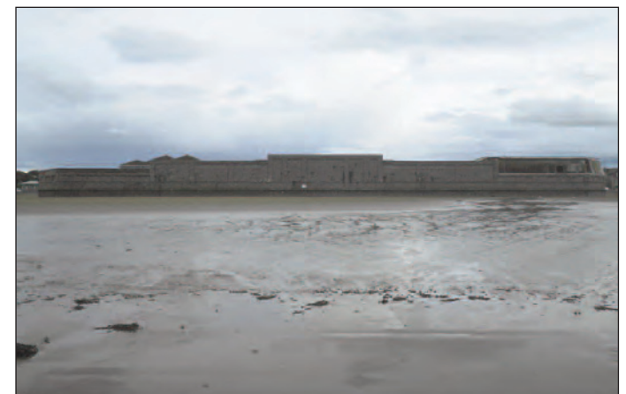
Plate 6 West-facing external elevation of the sea wall structure, looking east
