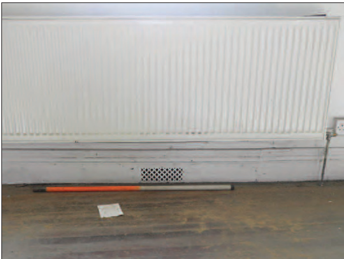
Plate 10 Original vent and skirting board of the central pavilion building, looking east
