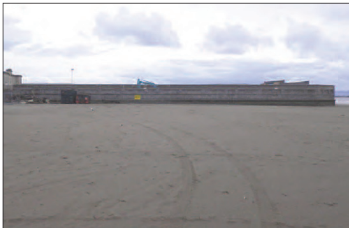
Plate 4 North-facing external elevation of the sea wall structure, looking south
