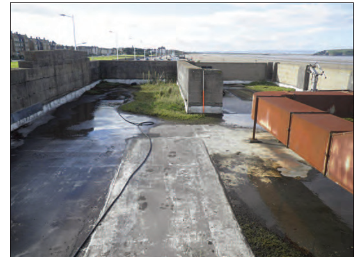
Plate 12 Roof of the south side wing, looking south
