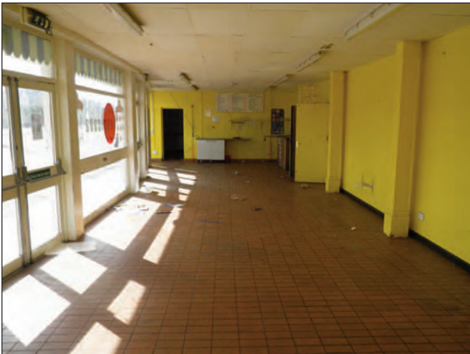
Plate 16 Shop space in the east side of the ground floor of the central pavilion building, looking south
