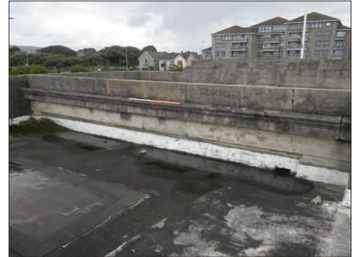
Plate 15 Pediment around the original edge of the roof, now within the flat roof space of the north side wing following a mid 20th-century addition, looking north-east
