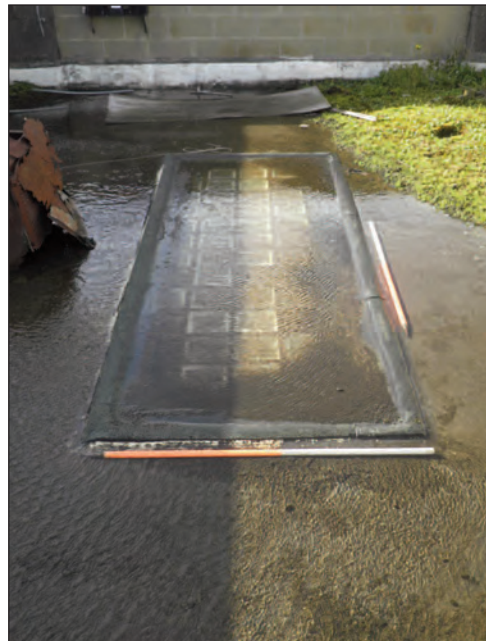
Plate 11 Roof light in the roof of the south side wing, looking south
