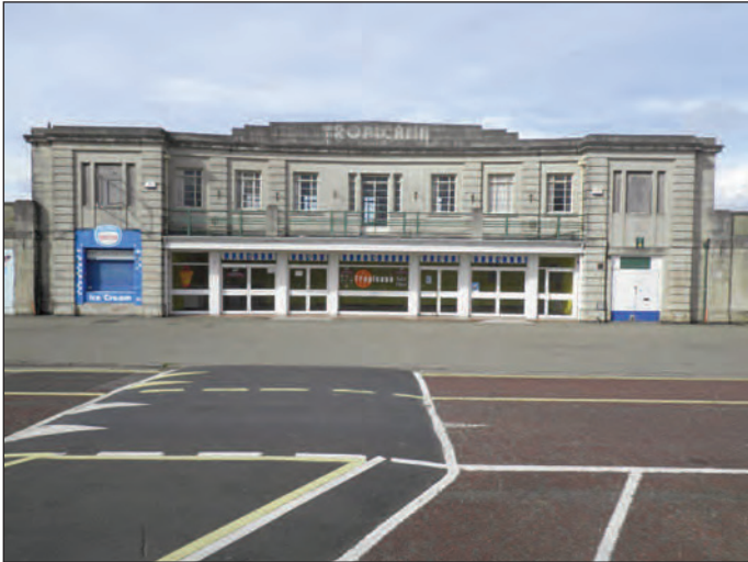
Plate 1 Front elevation of the central pavillion building, looking west
