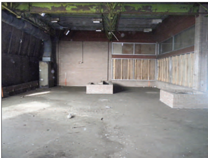
Plate 23 West room of the south range modern building, looking north
