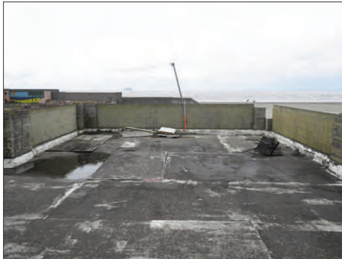
Plate 14 Roof of the north side wing, looking west
