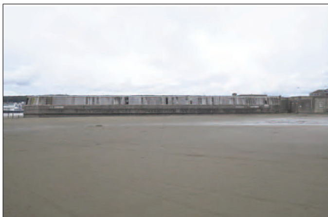
Plate 5 South-facing external elevation of the sea wall structure, looking north
