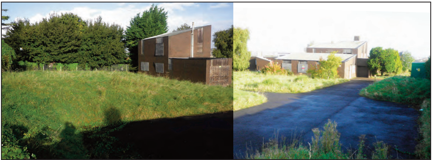
Plate 2 Southern extent of study area, looking north, substation to right of frame
