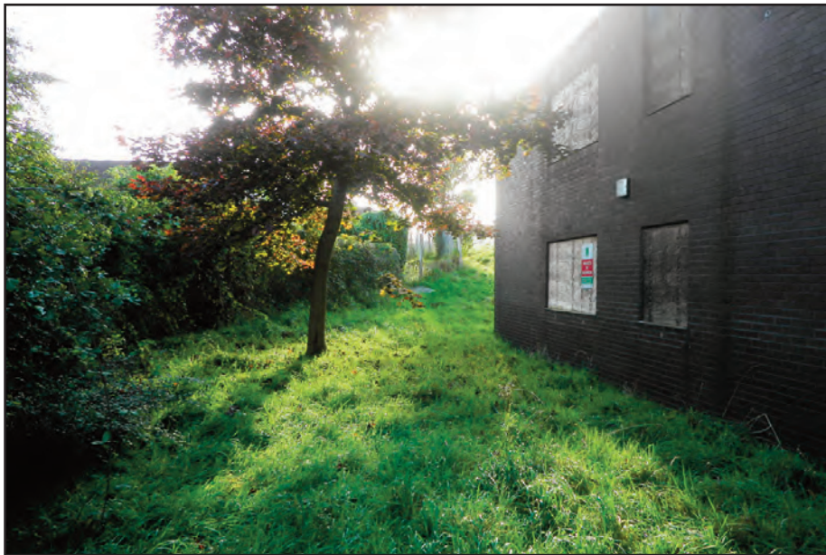
Plate 8 Northern extent of study area, looking east
