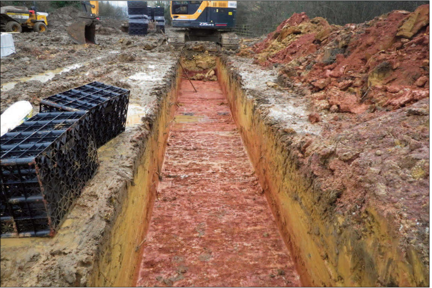
Plate 1 Drainage trench, looking east
