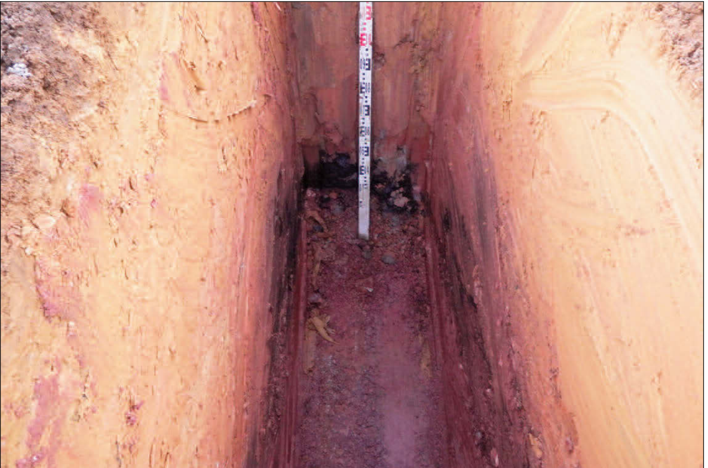
Plate 2 Foundation trench, looking west
