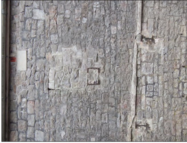
Plate 19 Blocking in south elevation of the principal building, looking north
