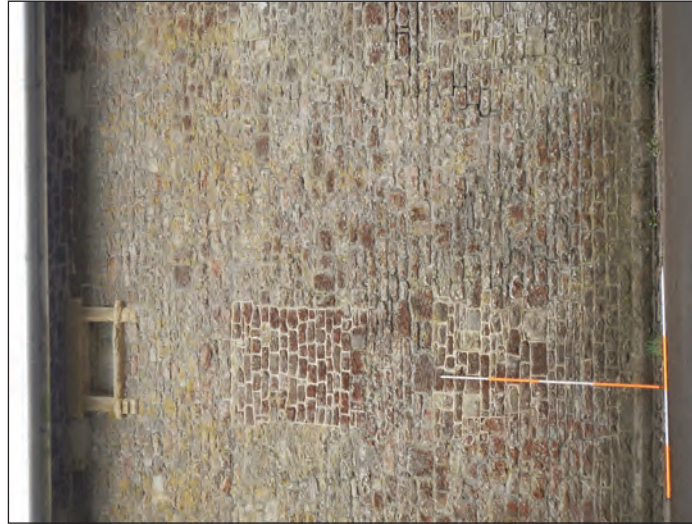
Plate 8 North elevation of the principal building, middle section, looking south
