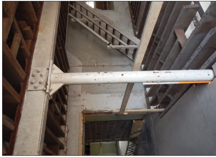
Plate 30 Column on the 2nd floor of the 1890s block, looking south-east
