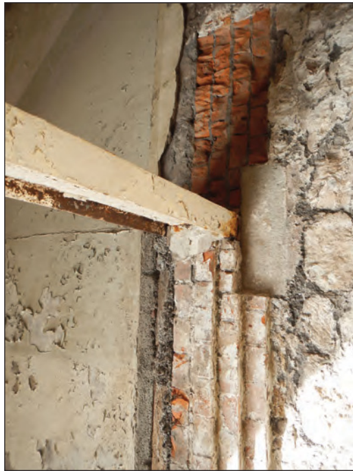
Plate 31 Iron beam set into north wall of the 1890s block, looking north
