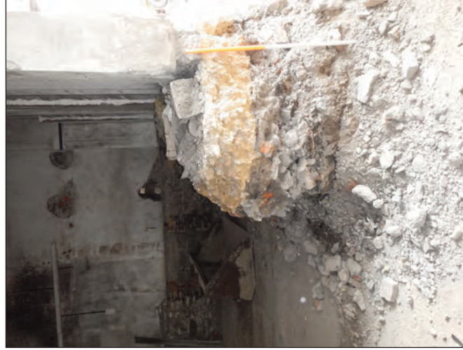
Plate 22 Remnant of raised floor, looking south
