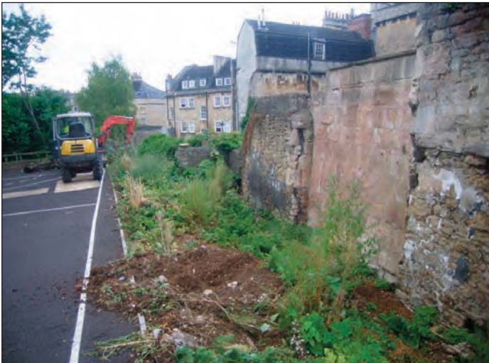
Plate 3 Looking south-west, alongside the eastern elevation of the boundary wall
