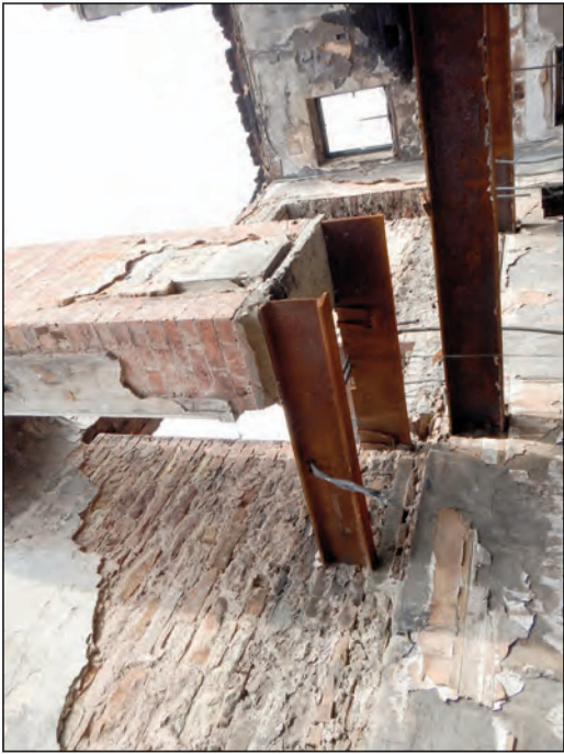
Plate 20 South wall, looking south-east, showing nails for keying plaster
