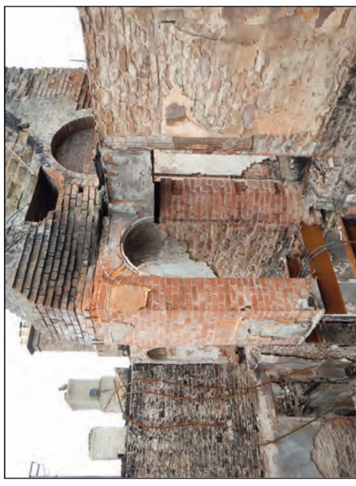
Plate 18 19th-century brick fireplace and arched doorway, looking north-east
