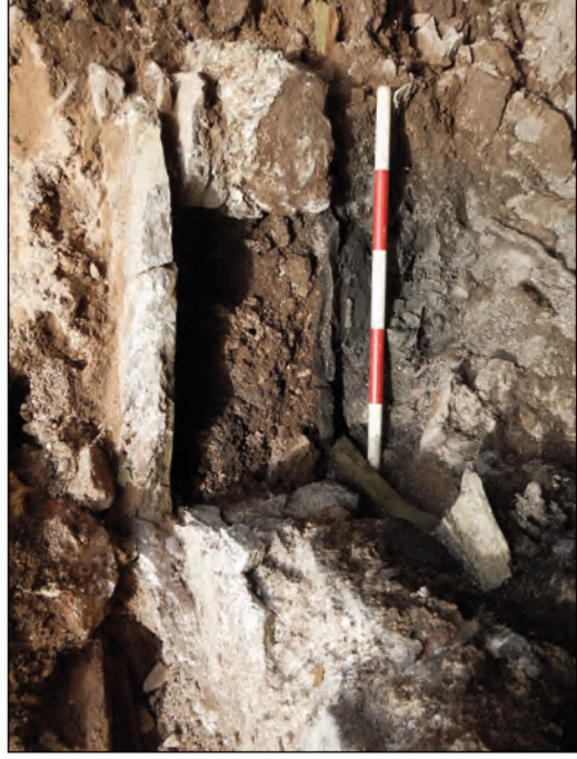
Plate 29 Drain 105 and later capping 107 in Trench 1, looking north
