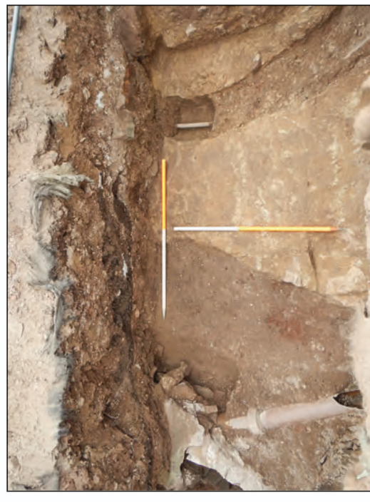
Plate 30 Lead water pipe 116 in Trench 1, looking south
