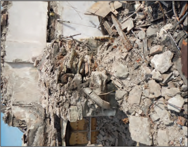
Plate 25 Partially demolished north-south dividing wall of the north wing, looking north
