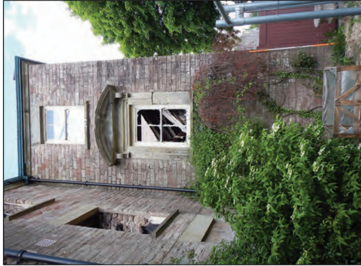
Plate 4 South elevation of the north wing of Newland House, looking north
