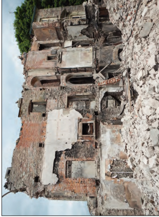
Plate 23 Original north wall, which became the central dividing wall following construction of the north wing, looking north-east
