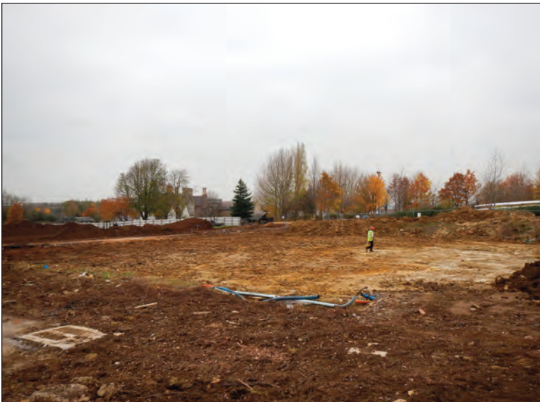
Plate 3 Area to the south-east of Wallscourt Farm, looking north-west
