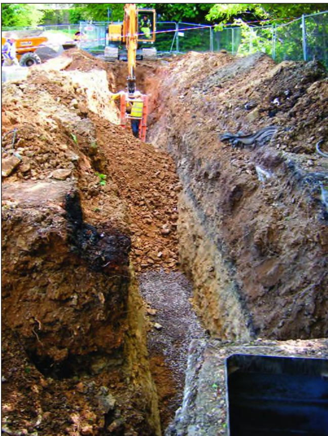
Plate 2 Representative view of sewer excavation
