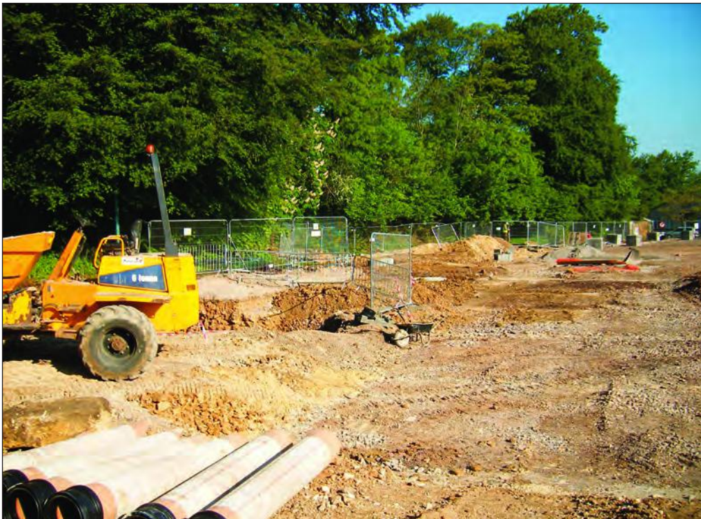
Plate 5 Partially backfilled sewer trench
