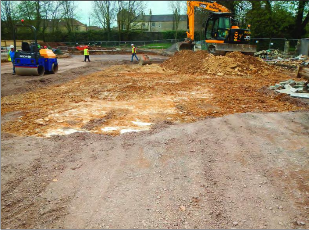
Plate 1 Site reduction and levelling for piling mat
