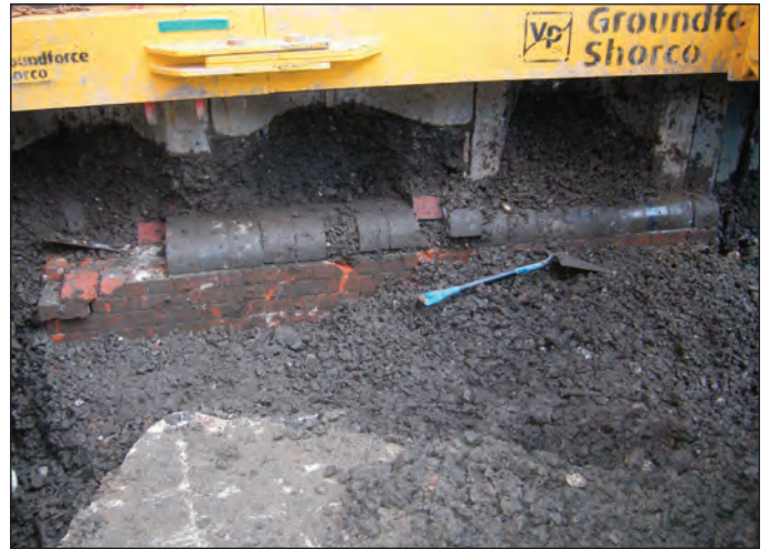
Plate 4 Top of original culvert, looking north-east
