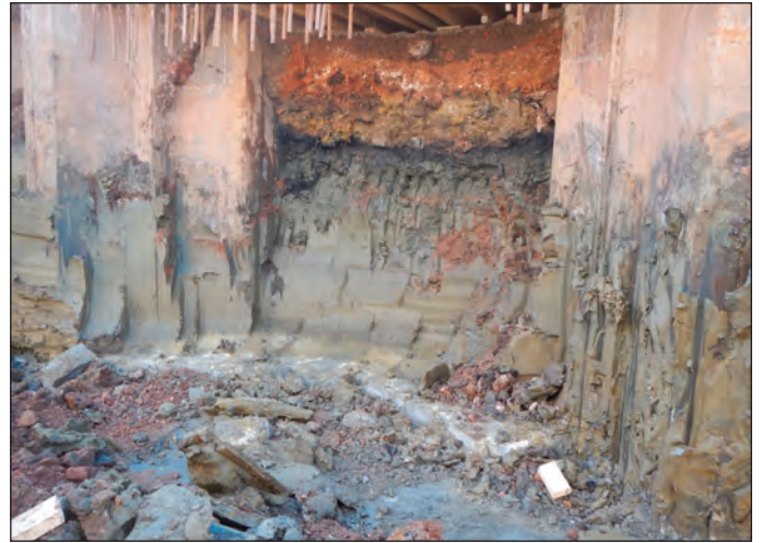
Plate 2 Representative section, looking south-west
