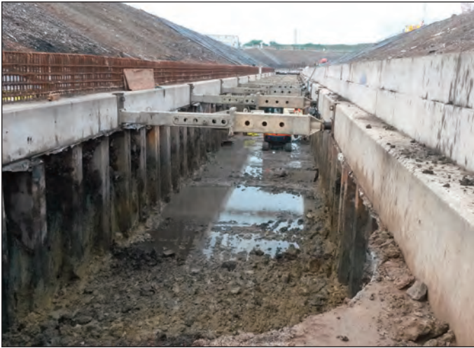
Plate 1 View along culvert, looking south-west
