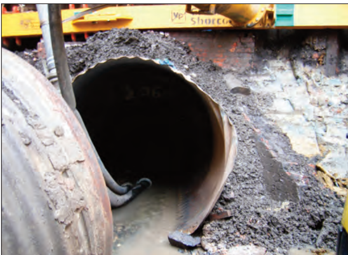
Plate 5 Corrugated steel pipe laid into brook and original culvert, looking north-east
