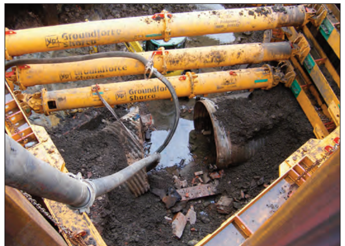
Plate 6 View down onto original culvert, looking south
