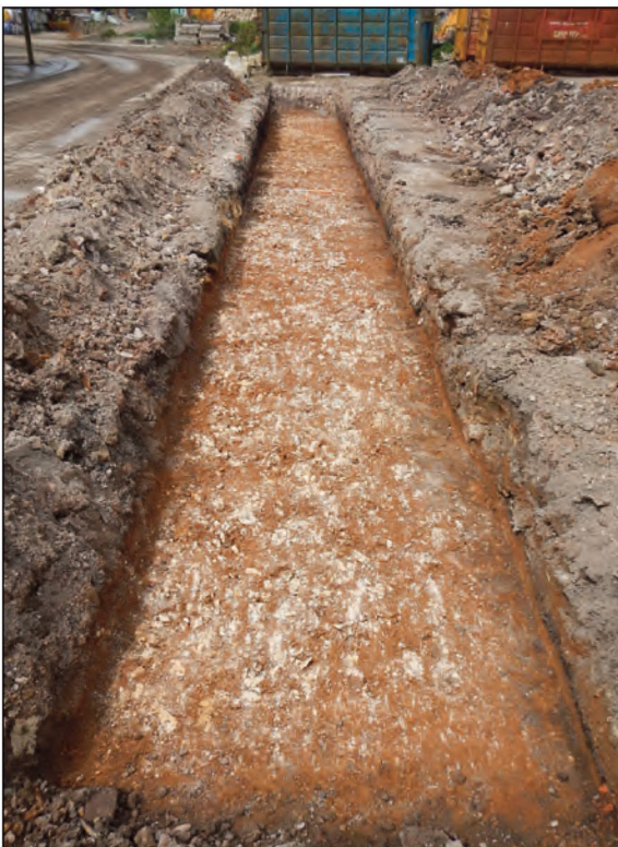
Plate 7 Trench 5, length of trench, looking north-west
