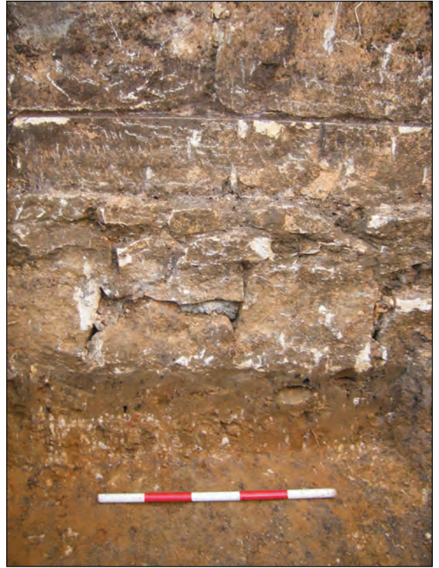
Plate 5 Representative section of south-eastern wall (113)
