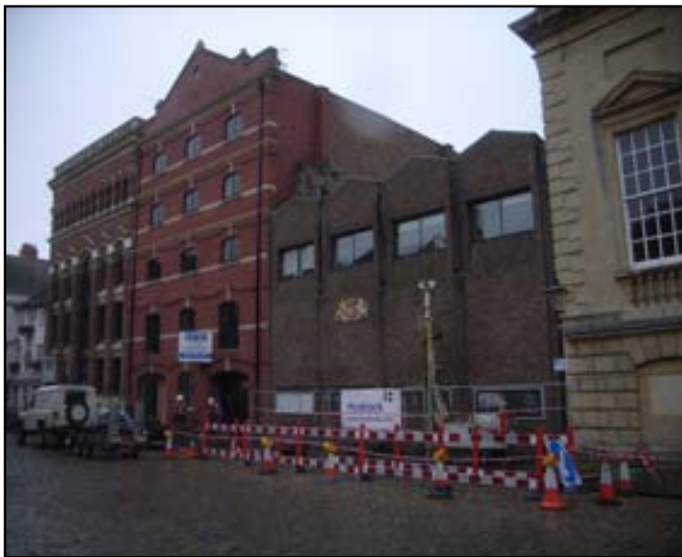
Plate 8 View of drilling rig outside the Theatre Royal, on the site of BH6
