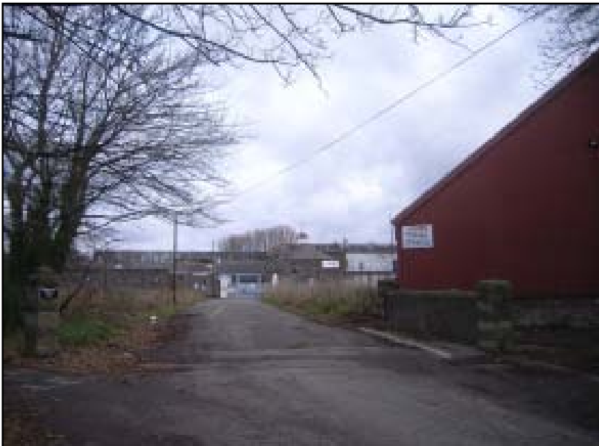
Plate 6 View east along the driveway towards the mill entrance
