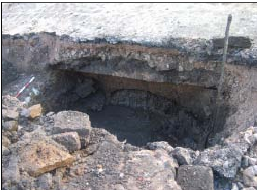
Plate 16 North-west facing section in TP 4. Left is wall 405, next to the culvert (404) entrance/exit
