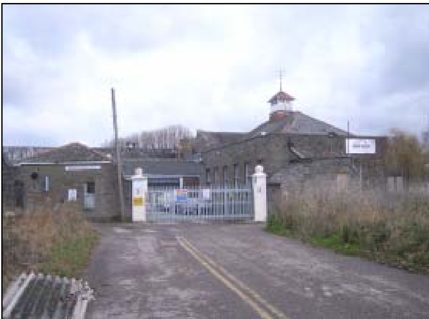
Plate 7 The main gates of Golden Valley Mills, the entrance flanked by the gatehouse (left) and the canteen (right)
