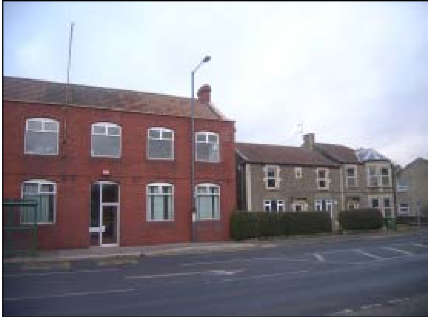
Plate 14 The Bath Road frontage of the Dacora Building (left) with Nos. 95 & 97 Bath Road next door (right)
