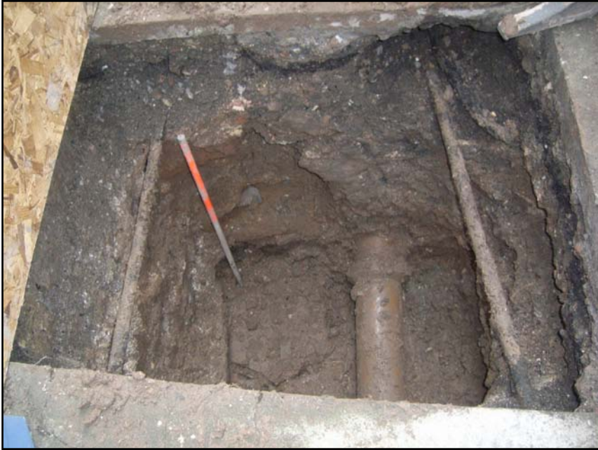
Plate 4 Long Walk service pit, looking west
