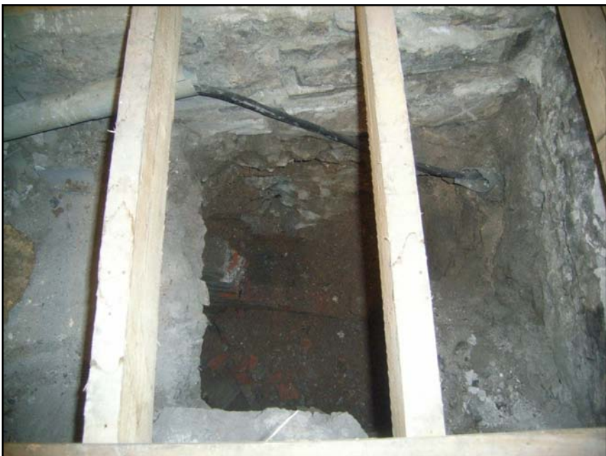
Plate 3 Vestry service pit after excavation, looking north
