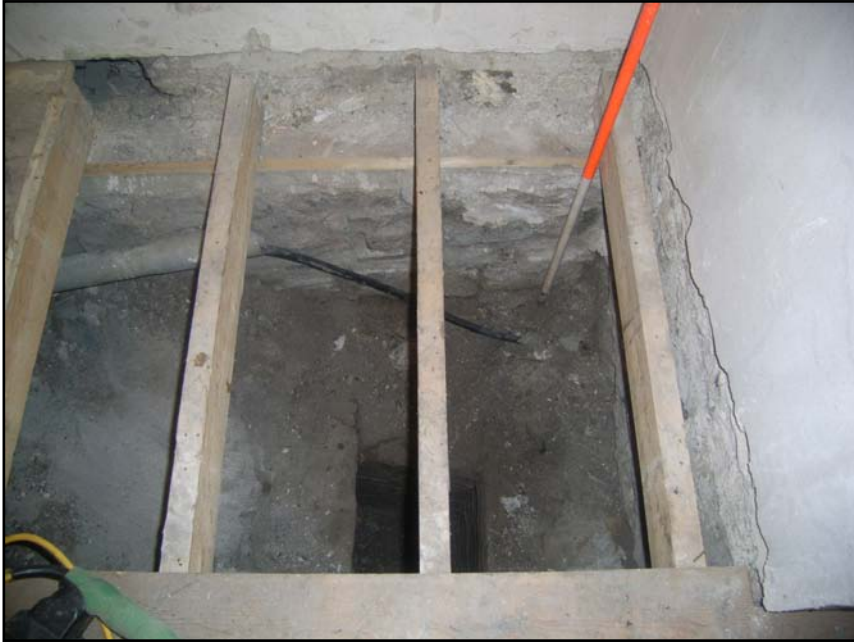
Plate 1 North-east vestry service pit, looking north during excavation
