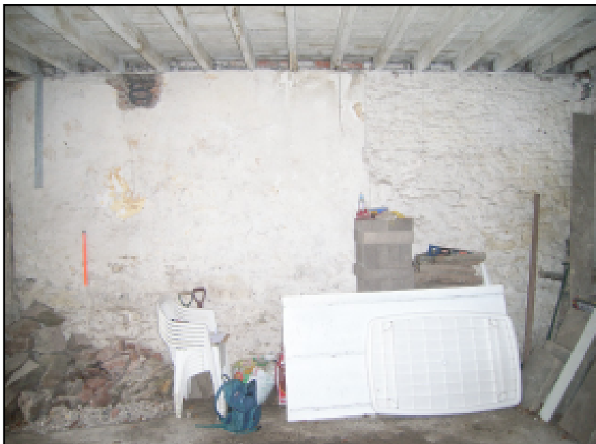
Plate 3 Internal view of the east elevation, from the west
