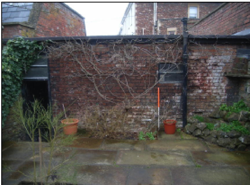
Plate 6 View of the rear elevation, from the south
