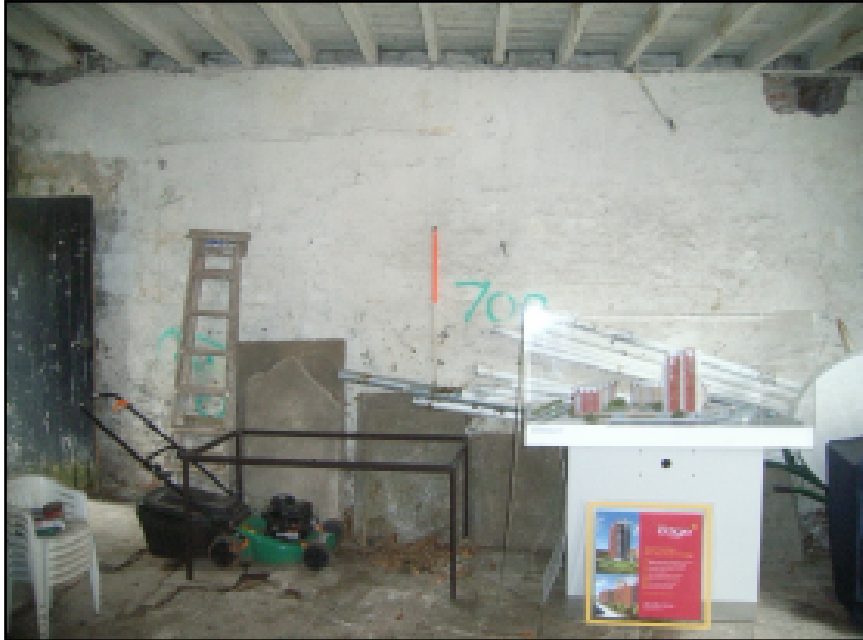
Plate 4 Internal view of the west elevation, from the east
