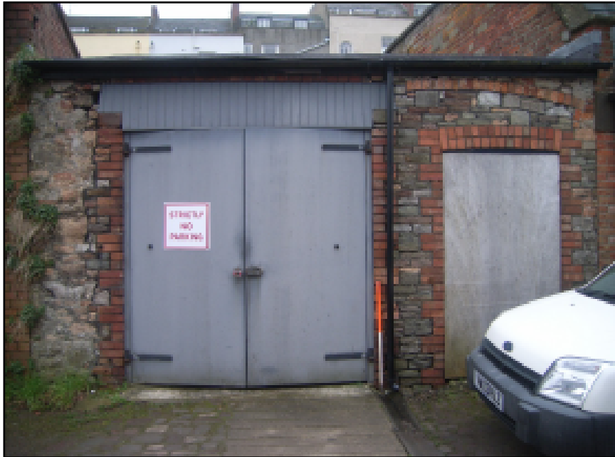
Plate 1 View of the front elevation, from the north
