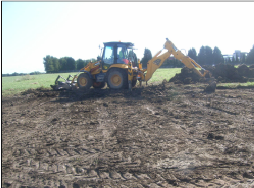
Plate 1 View of topsoil stripping
