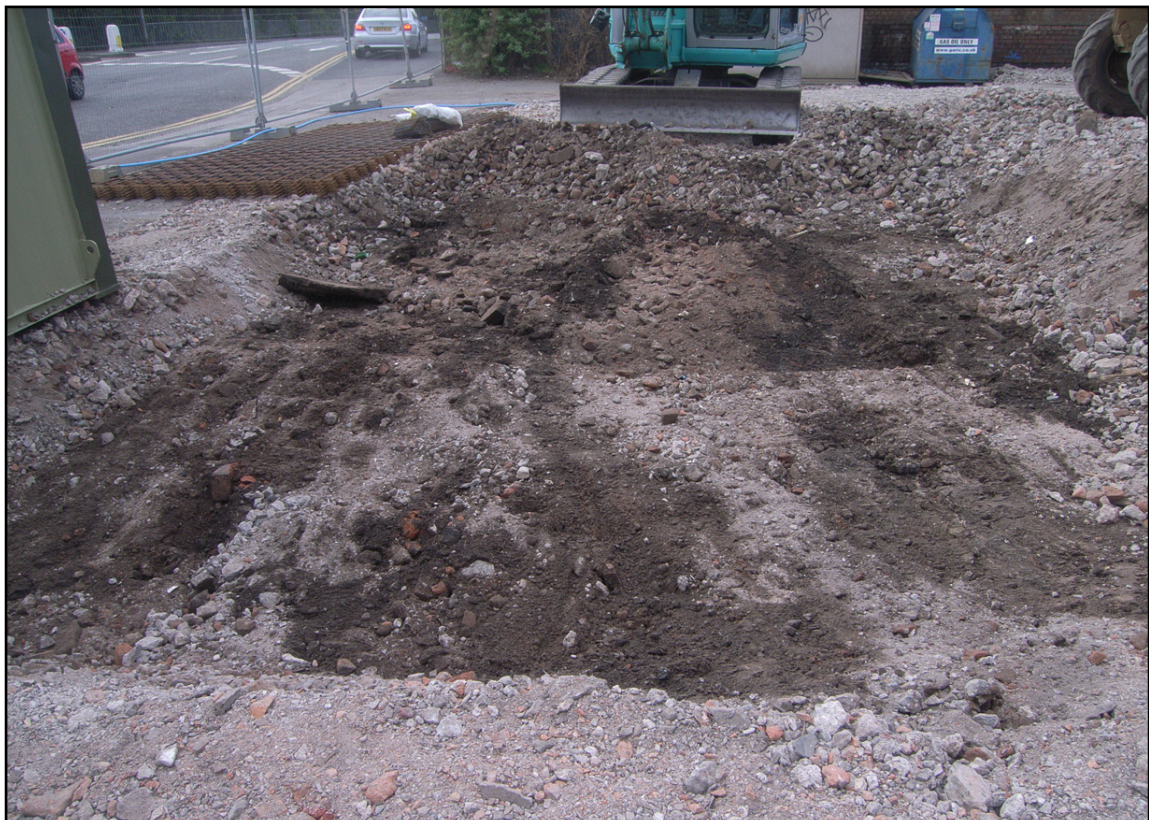
Plate 2 Trench 2 during excavation, looking south-west
