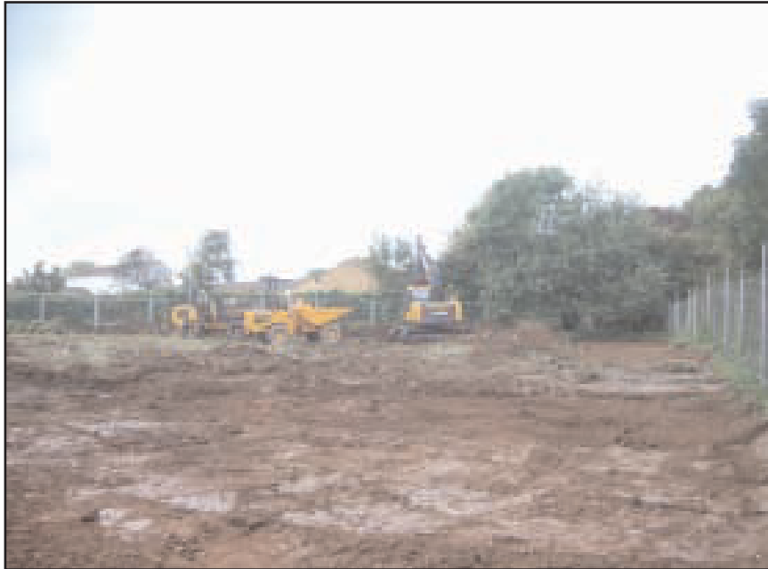
Plate 4 Main site strip in progress – looking north towards Stow House
