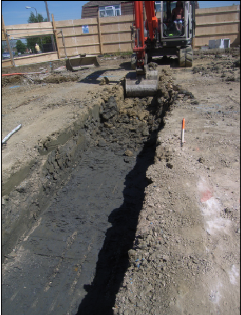
Plate 2 Excavation of foundation trenches in area B, looking north.
