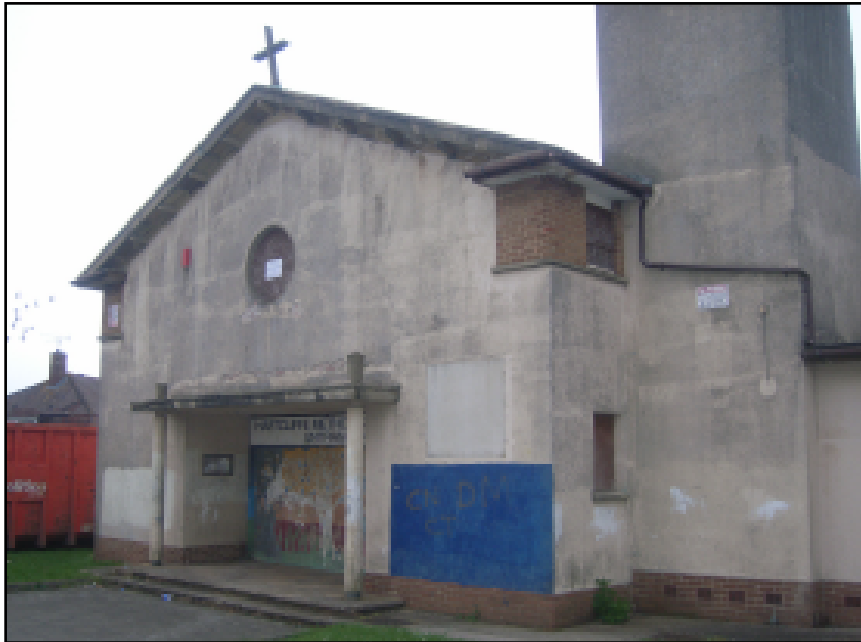
Plate 1 West front, from the south-west
