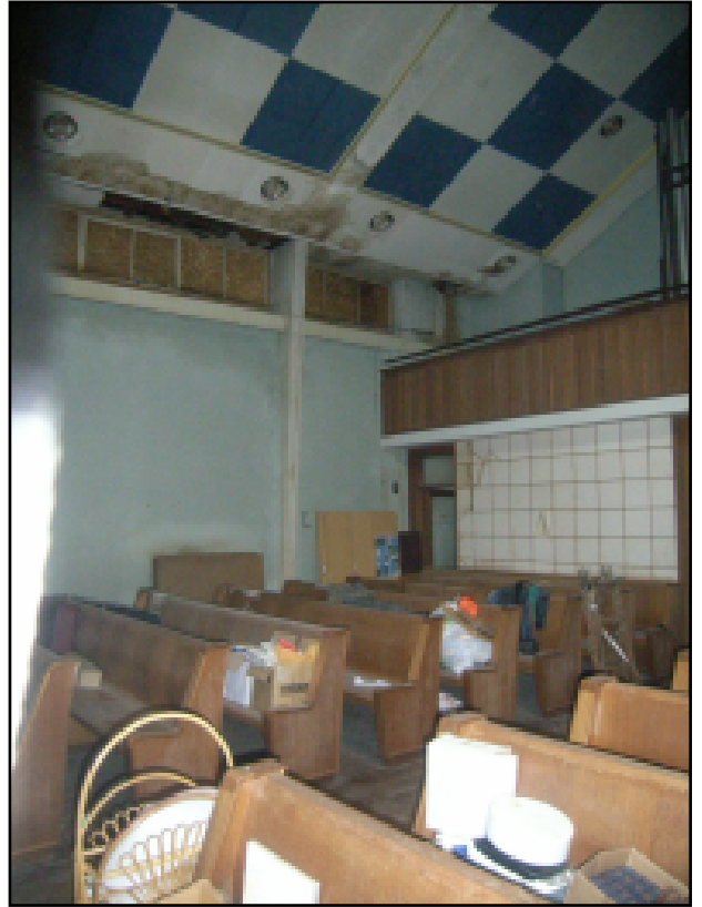
Plate 8 South-west corner of worship space
