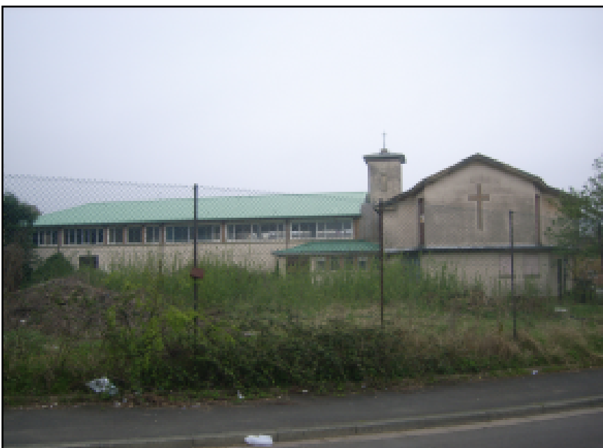
Plate 3 Church and hall from east
