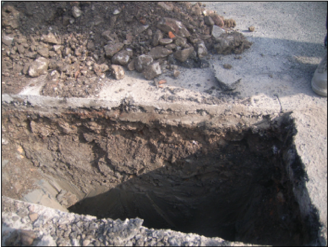
Plate 1 South-west facing section of Test Pit 1
