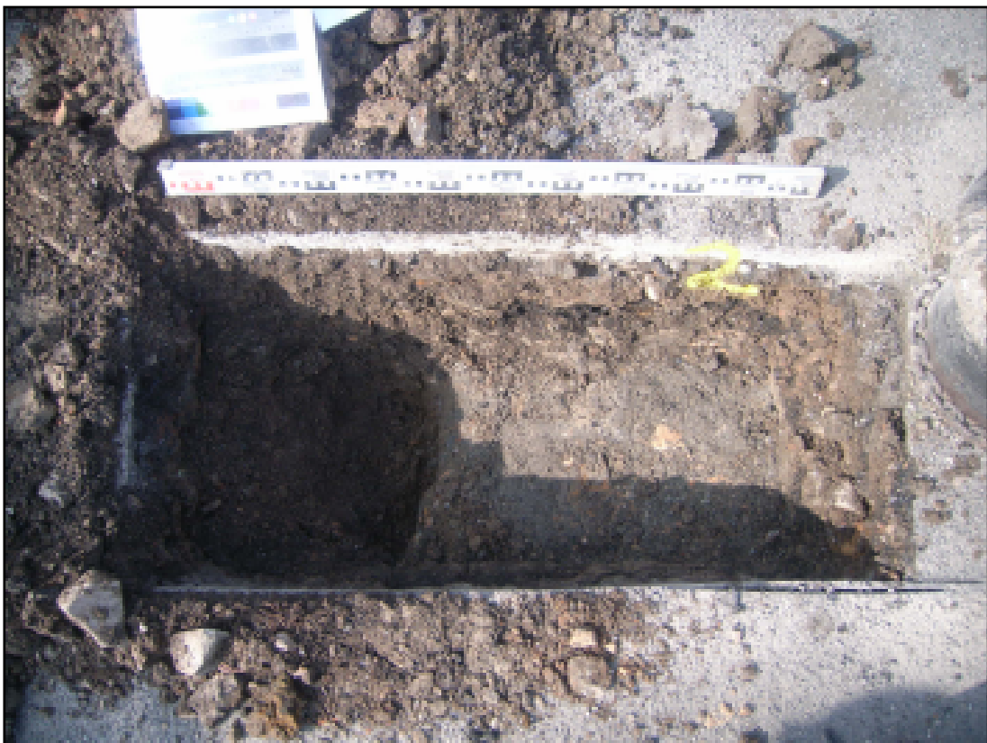
Plate 2 View of mooring post footing, Test Pit 2
