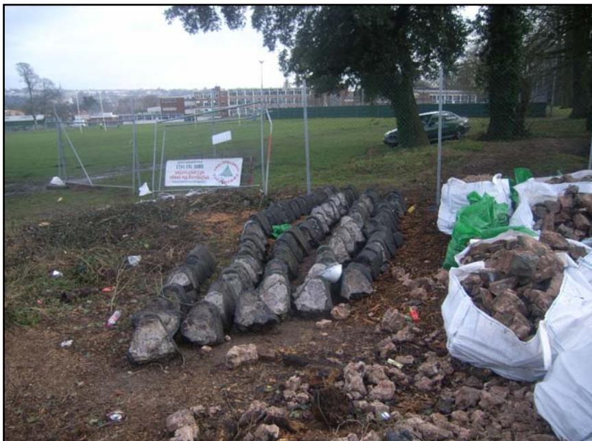
Plate 2 View of bagged-up stone and set-aside slag coping-stones during dismantling phase
