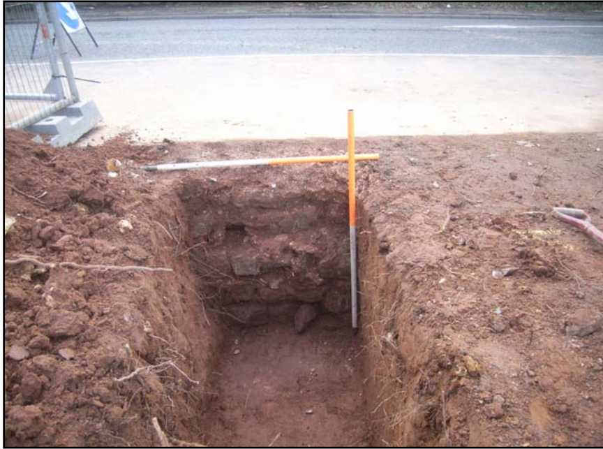
Plate 3 General view of sondage excavated on northern side of boundary wall following dismantling phase, from the north
