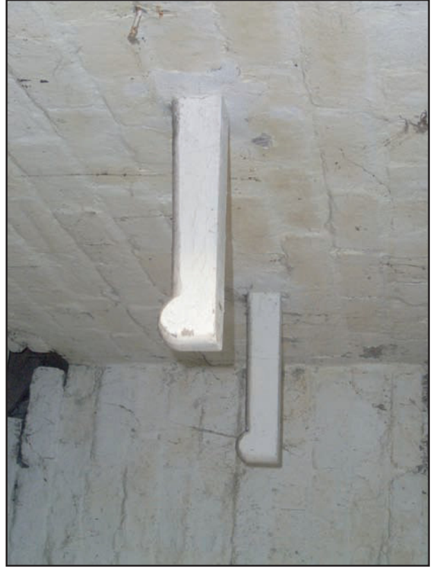
Plate 22 Wooden pegs in stable wall
