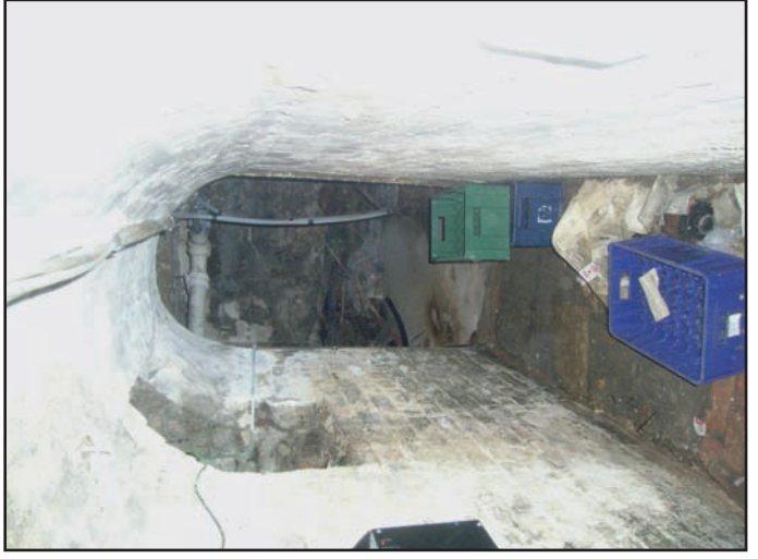
Plate 16 Cellar passage looking south-west, with vent on left
