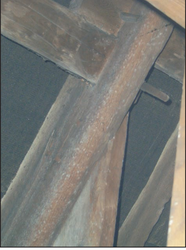
Plate 27 Detail of rear roof, as seen from bathroom hatch
