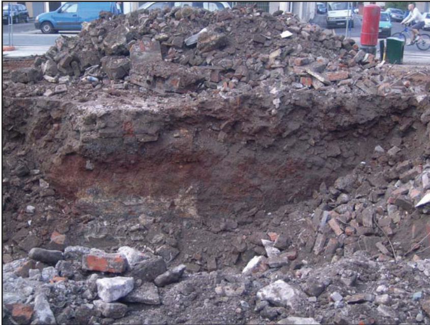
Plate 4 The section revealed after the removal of the north-west wall of cellar 015, looking north-west
