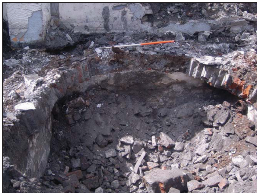
Plate 3 The barrel-vaulted roof of cellar during excavation, looking south-west
