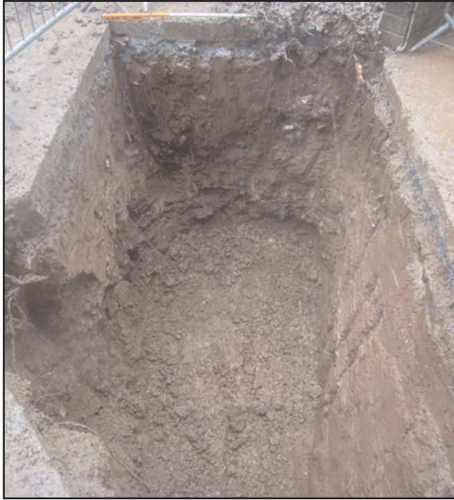
Plate 4 Pile-cap box D at the completion of excavation
