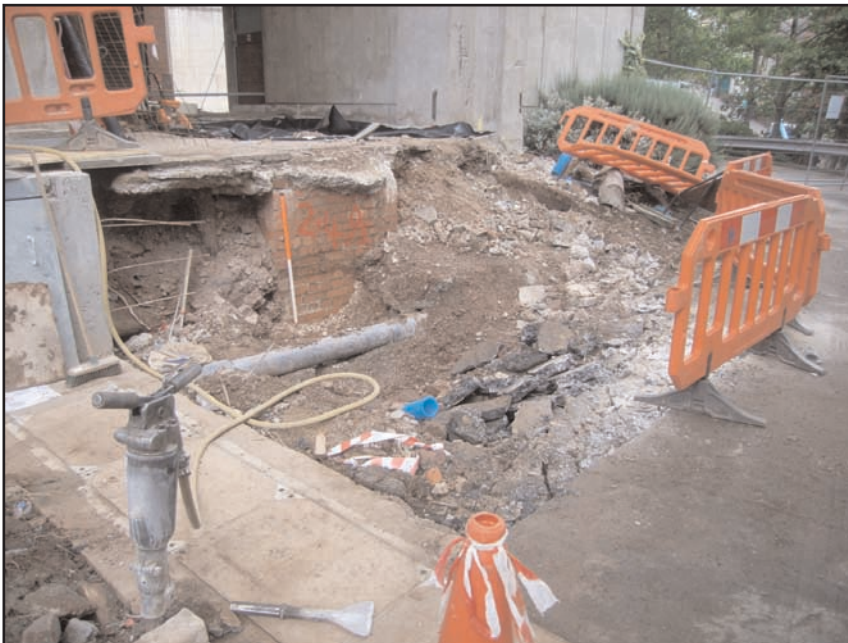
Plate 2 Reduced level excavation in area of Service Trench 200
