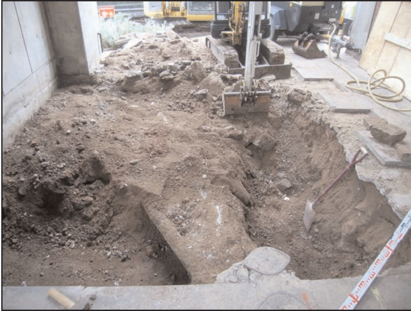
Plate 1 General view of Service Trench 100 after excavation
