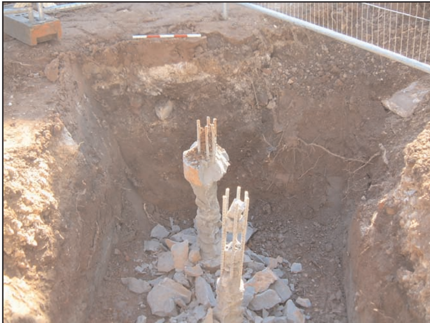
Plate 5 Pile-cap box H at the completion of excavation
